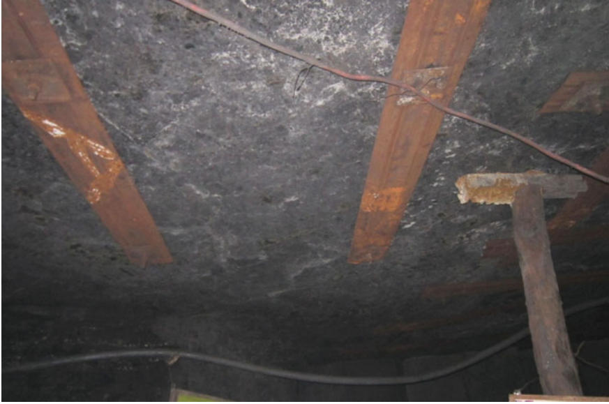
Fig. 14 The rock bolts along with W-straps support system
