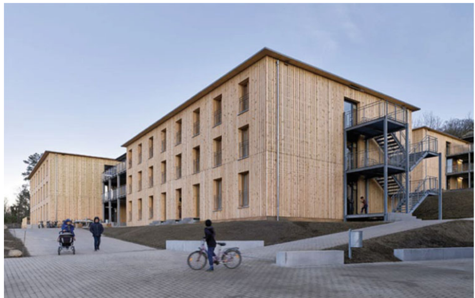
Fig. 7 The efforts of Three separately commissioned architecture firms collaborating to develop a modular system using wood as the material for flexible reuse and promotion of a regional supply chain sustainability. Three projects housing between 100 and 300 asylum seekers have each been completed within less than a year. Source Spaces of Migration: Architecture for Refugees (2018)
