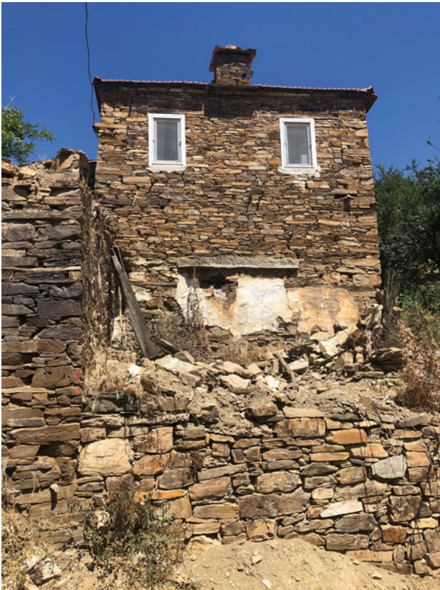
Fig. 8 Material change in the windows of the traditional residential building in Dernekli Village. 2020
