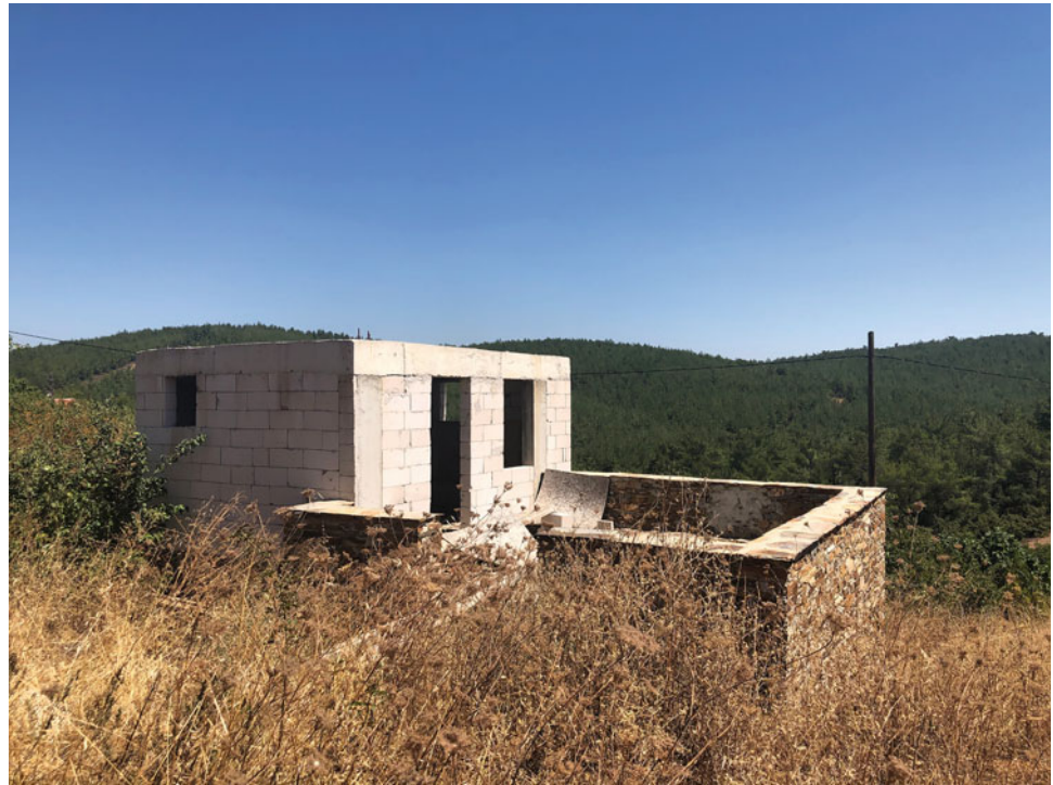
Fig. 21 New construction with existing material and contemporary materials over the remains
