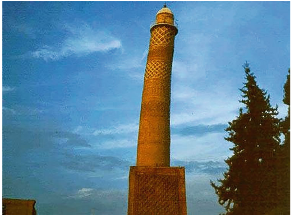
Fig. 5 This did not happen in the Al-Hadba minaret, because the land of Mosul was rocky and hard, and the curve became in the body (The minaret of Humpback in Mosul)
