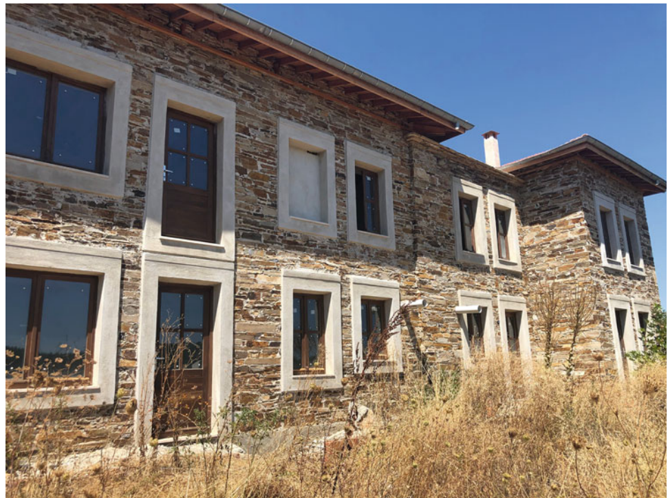
Fig. 23 New construction over the remains
