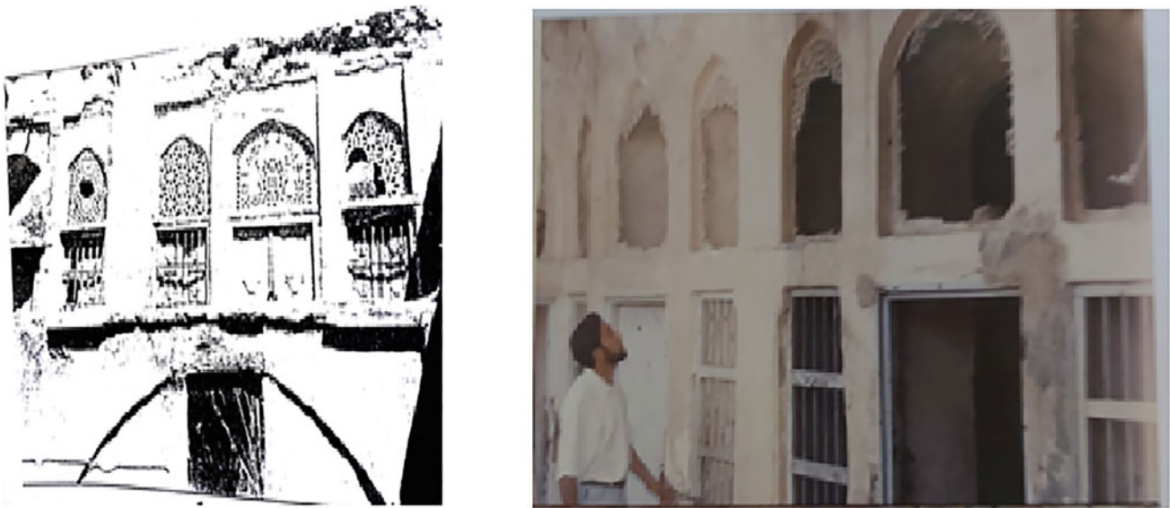
Fig. 2 The internal façades of the traditional heritage houses in Samarra
