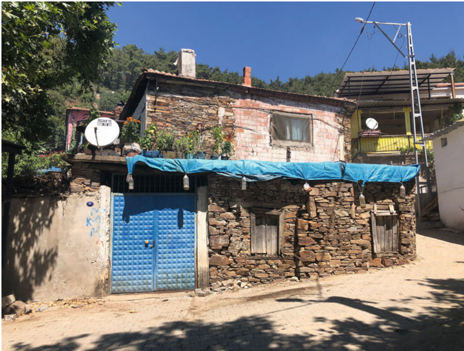
Fig. 7 Unqualified intervention with brick material in the traditional housing building of Dernekli Village. 2020
