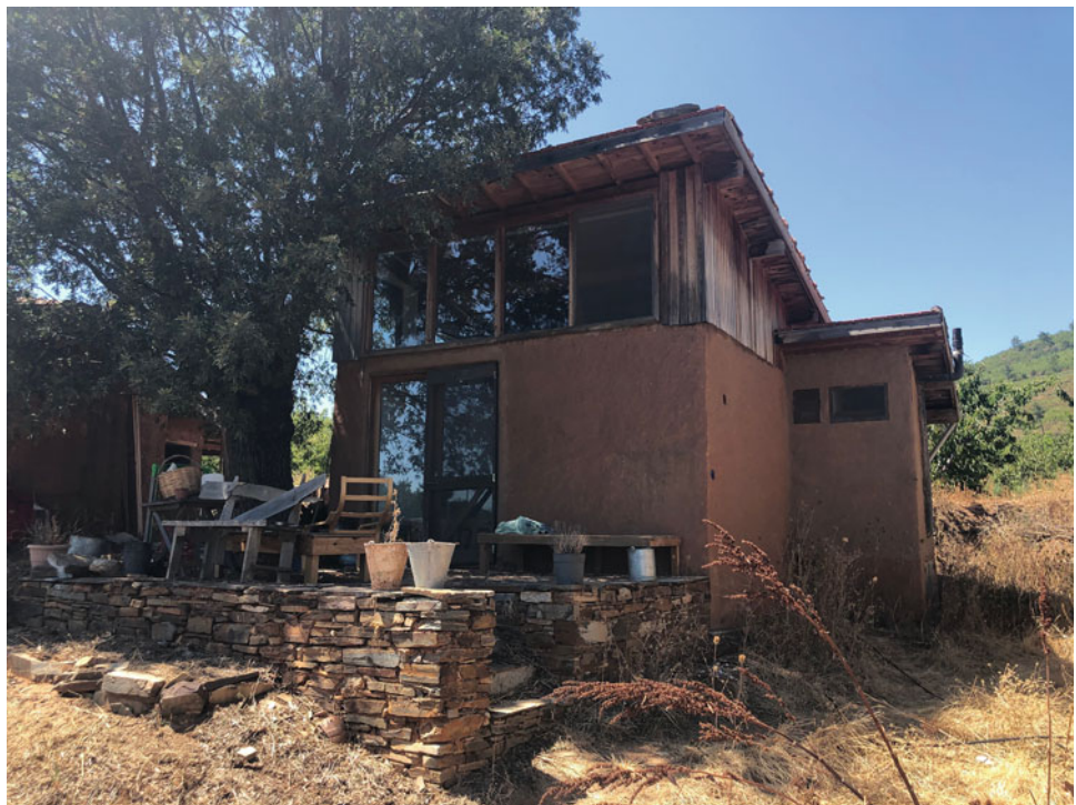
Fig. 20 New construction application with the masonry soil technique
