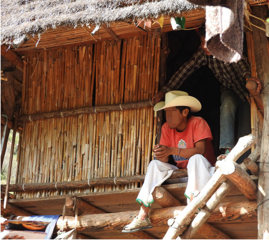
Fig. 23 Trolley where they guard the harvested corn, the walls are built with otate ( Otate sp.). (Photo by: Mara Ximena Haro-Luna)
