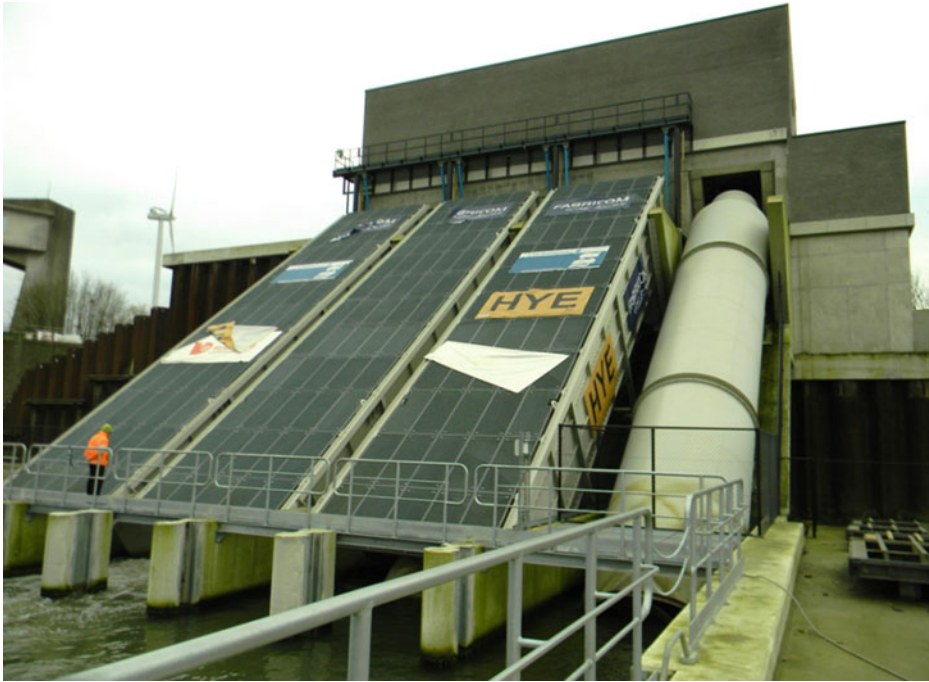
Fig. 11.1 The hydropower station of Ham (Belgium), equipped with three Archimedes hydrodynamic screws (on the left; the cover does not turn with the screw and is fixed; the screws can pump water and generate power as turbine), and one true Archimedean screw (on the right, the cover is fixed to the screw and turns with it; this screw can only pump water)
