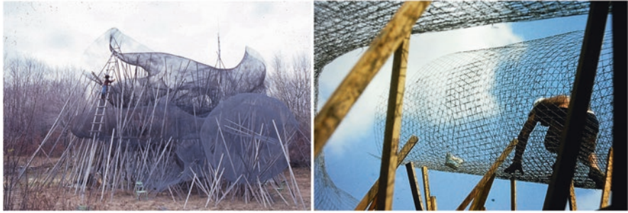
Fig. 8.6 Liberty Rural Community Centre , Parksville (1976–1979). On the left, view of the structure; on the right, Giorgini walking on the structure for manually modelling the meshes (Courtesy B.A.Co. -Vittorio Giorgini Archive)
