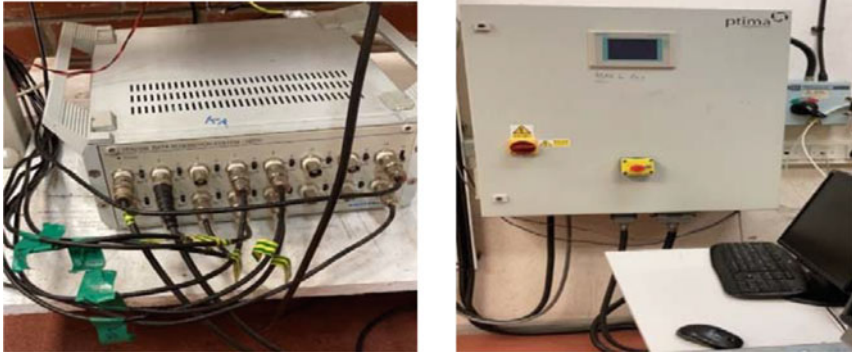
Fig. 5 Data acquisition system (left) and generator controller (Right)
