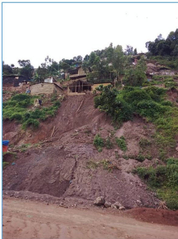
Fig. 12.1 Steep slope of Bukavu, where terraces built to accommodate new houses reinforce the risk of landslides (© HARISSA Citizen Observers network—RMCA, December 2020)
