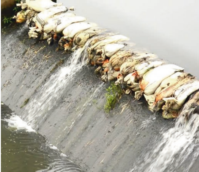
Fig. 9.2 Sandbags to prevent floods
