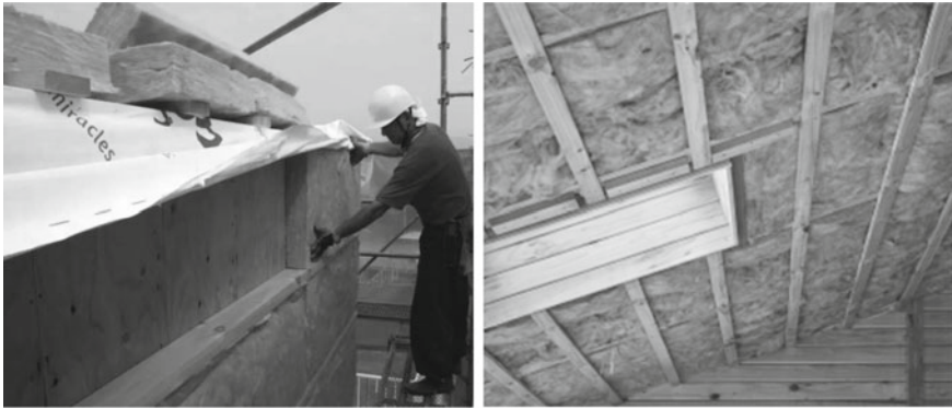
Fig. 5.9 Glass wool insulation installation
