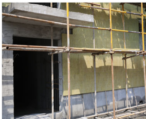
(b) Wall insulation
