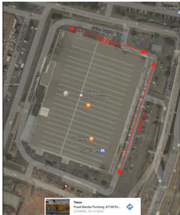
Fig. 4.30 Roof top view of an actual hypermarket (with GPS coordinates) (Source Google Map)
