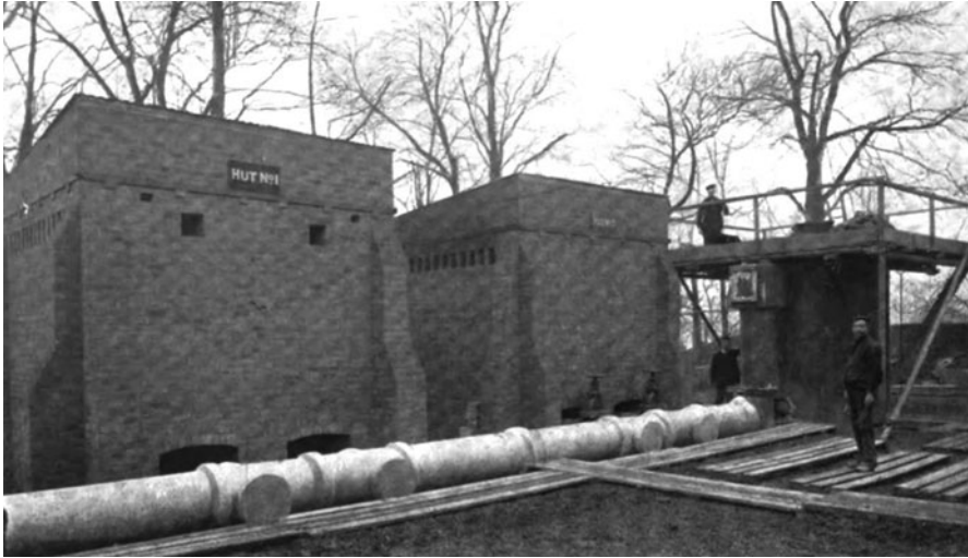
Fig. 2.1 The test huts at the first UK fire testing station, built in London in 1899 by Sir Edwin Sachs
