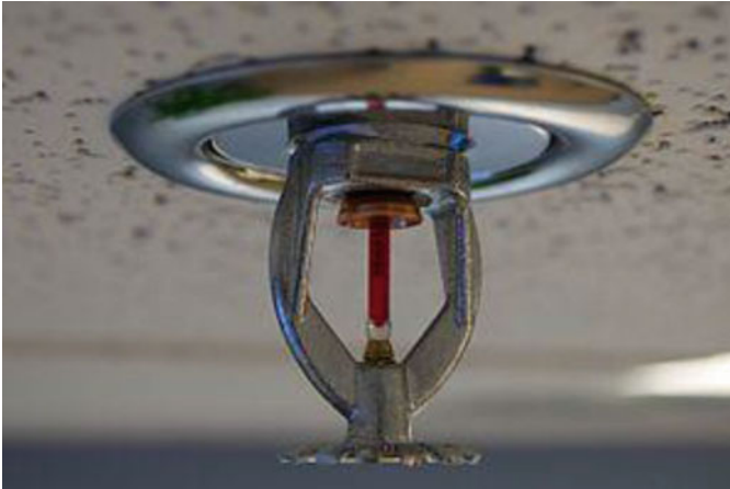
Fig. 5.1 Fire sprinkler head [2]
