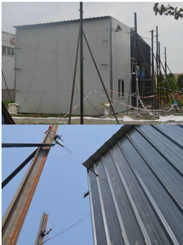
Fig. 13.22 Mounting of LVDT on the structure
