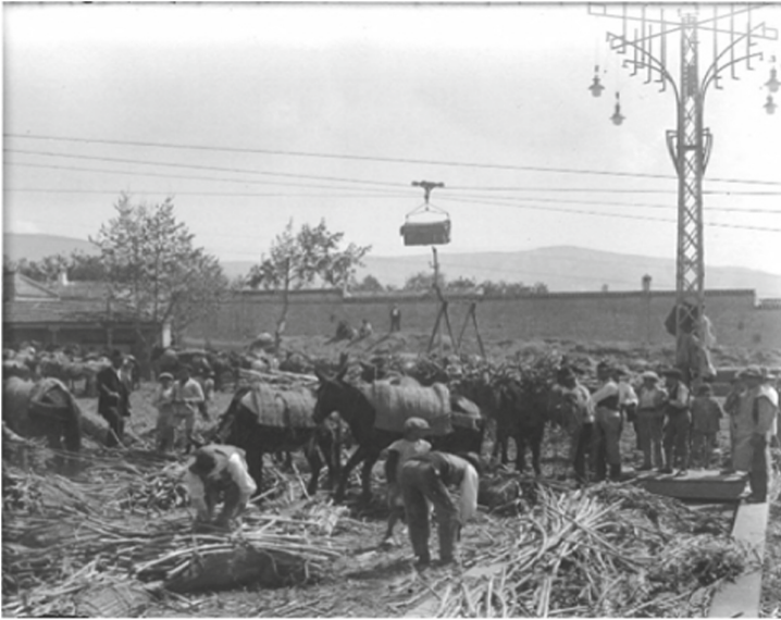
Fig. 2. Cane square and overhead cable laying [7]
