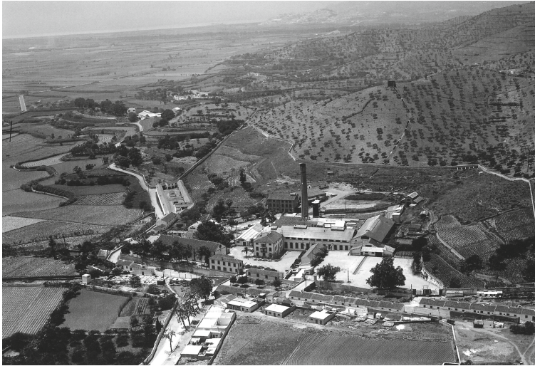
Fig. 1. Aerial overview. Azucarera del Pilar [5]
