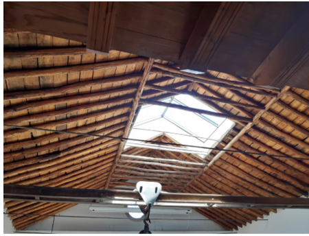
Fig. 7. Detail of the wooden roof and the skylight. (owner’s collection).
