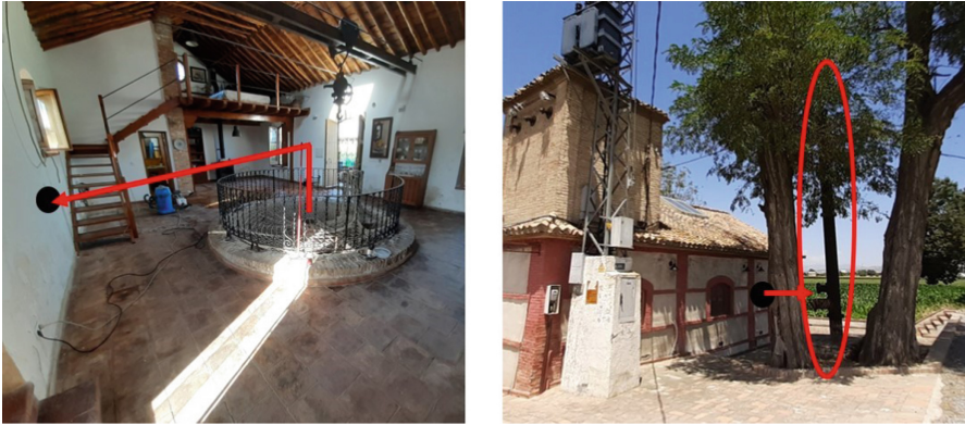
Fig. 13. Direction of the pipe a) inside the building and b) outside the building
