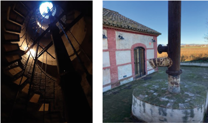
Fig. 12. The extraction pipe of the well a) seen from the bottom b) outside de house. (particular collection).
