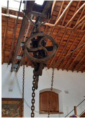
Fig. 9. Clamped beam to support the bridge crane. (particular collection).
