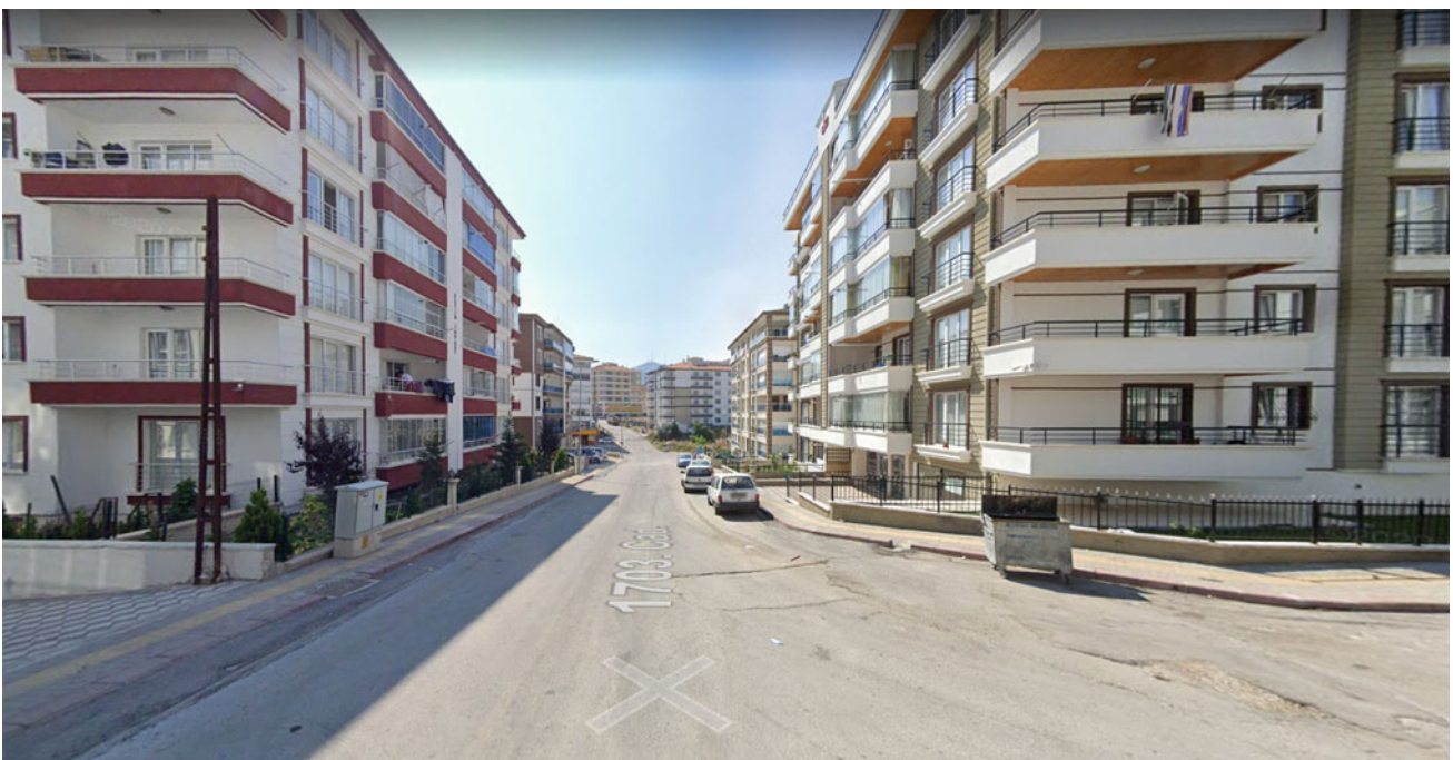
Fig. 23 The new urban regeneration building. Photograph taken from Google Map
