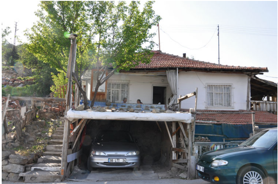
Fig. 18 A squatter housing-unit in Feridun Çelik. Photograph taken by the author
