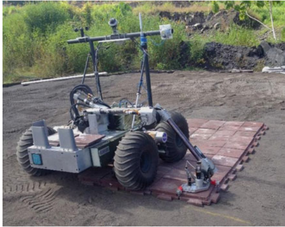
Fig. 12.20 PISCES Rover Helelani assembling interlocking pavers made with sintered Hawaiian Basalt (Romo et al. 2018)
