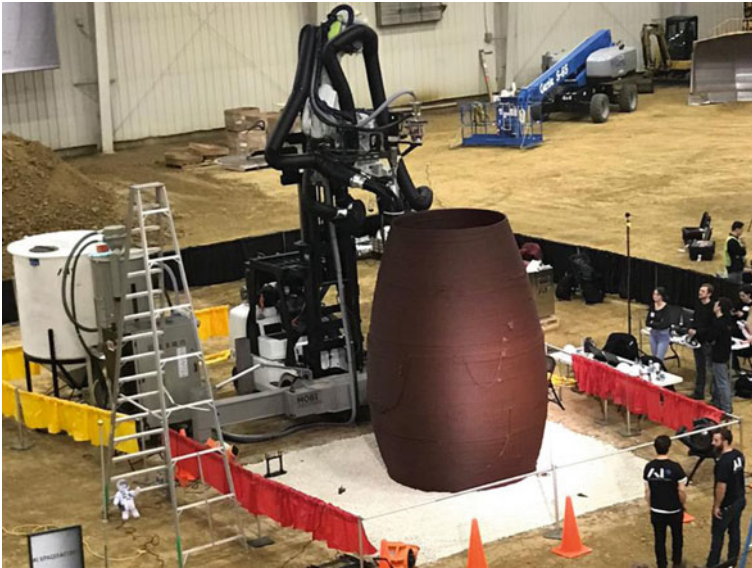
Fig. 11.14 A PLA thermoplastic polymer/regolith material being 3D printed at the NASA Centennial Challenge competition for “3D Printing a + Habitat” by the winners: A.I. Space Factory. Credit NASA
