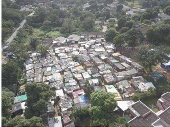
Fig. 1 Aerial view of the Havelock settlement and the river affecting dwellings
