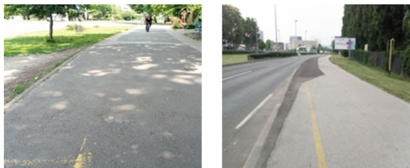
a) Unmarked bicycle path (worn-out markings)
