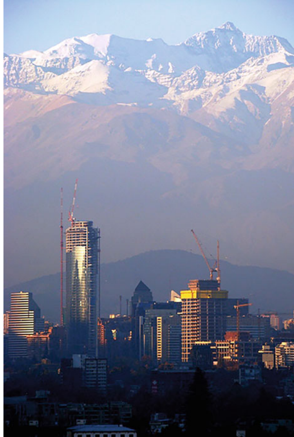
Fig. 4 Titanium La Portada under construction, Santiago, Chile; photo © 2020 Cristobal Barra, used with permission
