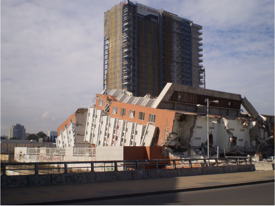
Fig. 5 Concepcion, Chile, after the earthquake in 2010; photo © 2020 Patricio Duran
