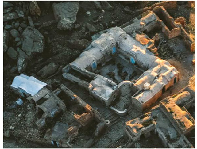
Fig. 18 The house after rehabilitation
