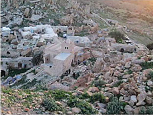
Fig. 4 Current photo showing the degradation
