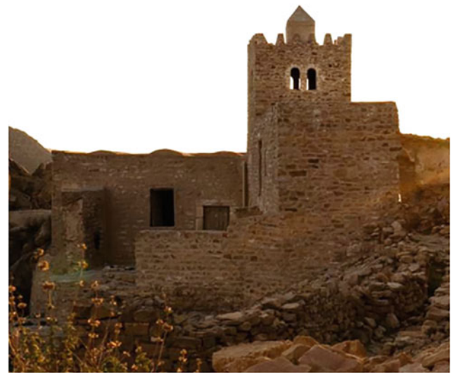
Fig. 6 The mosque after restoration
