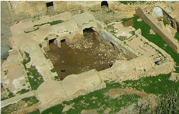
Fig. 16 Abandoned construction that requires general maintenance to preserve the original architectural aspect
