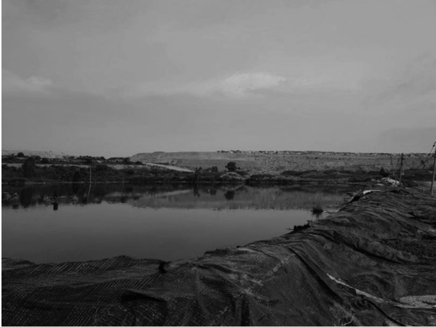
Fig. 8.7 The leachate collection pond at the Pulau Burung landfill site (PLBS), Penang, Malaysia
