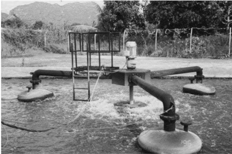
Fig. 8.11 A typical aerated lagoon
