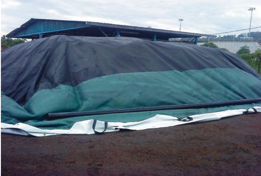
Fig. 7.30 Waste heaps covered with geotextile
