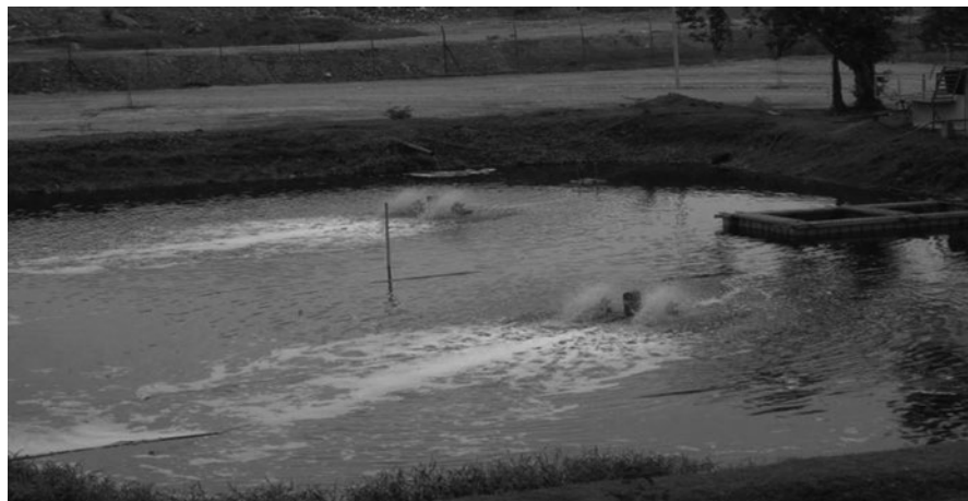
Fig. 8.6 Ampong Jajar Landfill Site Leachate Collection Pond, Penang, Malaysia
