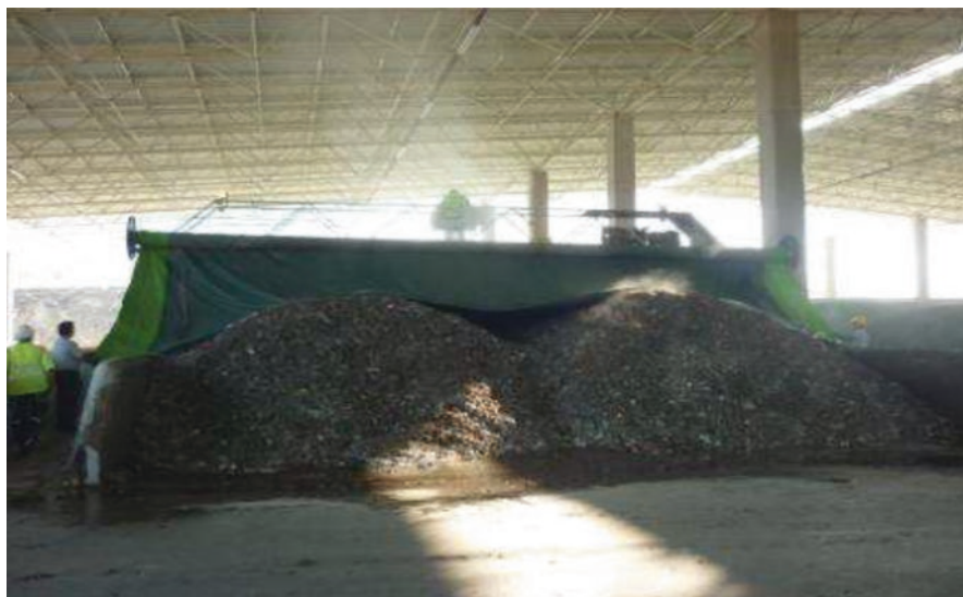
Fig. 7.33 Automatic machine to remove the geotextile membrane
