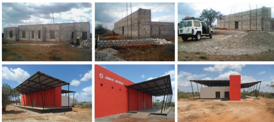
Fig. 14.3 Chakama dispensary building site
