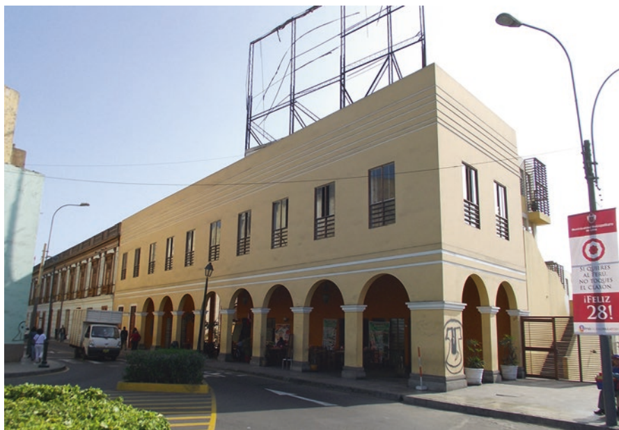
Fig. 10.10 Insertion of the La Muralla Housing Complex in the pre-existing urban context. Source: Chapter’s author Collection
