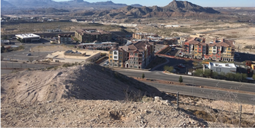
Fig. 21.8 Project Site in El Paso, Texas (Photo Courtesy AGENCY Architecture LLC)
