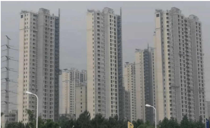
Fig. 9.9 Material use: more steel and reinforced concrete for construction of new high-rise buildings in Ningbo, China (Source: Ali Cheshmehzangi)
