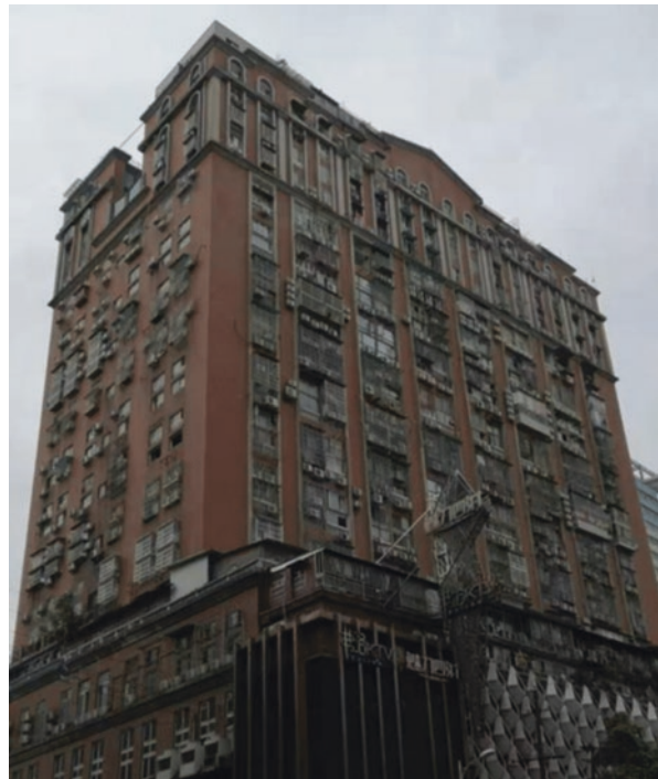
Fig. 9.5 Building services: air conditioning units as one of the main building services visible on the building façade in Changsha, China (top), and on the roofs in Osaka, Japan (bottom) (Source: Ali Cheshmehzangi)
