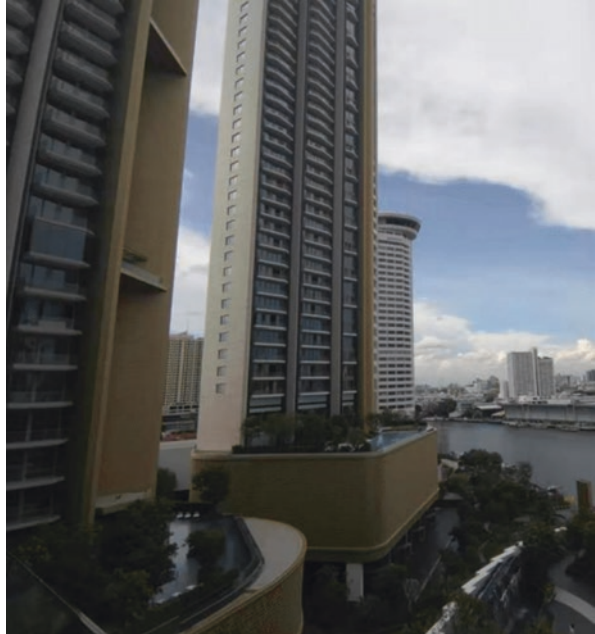
Fig. 9.11 Design and planning paradigms: a new high-end and high-rise residential compound in hot and humid Bangkok, Thailand, incorporating some key design features but still with a large ratio of glazed facades (top) and a low-to-midrise residential compound in hot and dry Shiraz, Iran, incorporating scale and façade configuration, but still with little consideration of spatial strategies for green infrastructure integration (bottom) (Source: Ali Cheshmehzangi)
