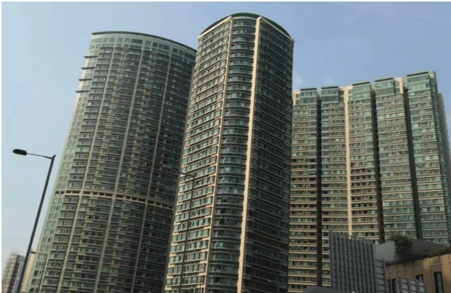
Fig. 9.7 Façade design: large ratio of glazed facades for a cluster of residential towers in Hong Kong, China, with extreme hot and humid climatic conditions and with a high cooling demand (Source: Ali Cheshmehzangi)
