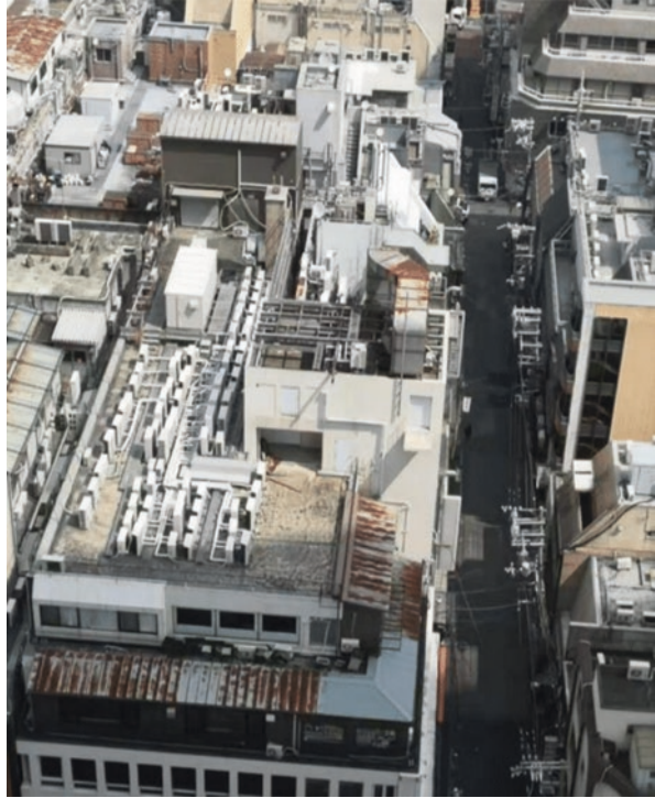
Fig. 9.6 Building services: air conditioning units as one of the main building services visible on the building façade in Changsha, China (top), and on the roofs in Osaka, Japan (bottom) (Source: Ali Cheshmehzangi)
