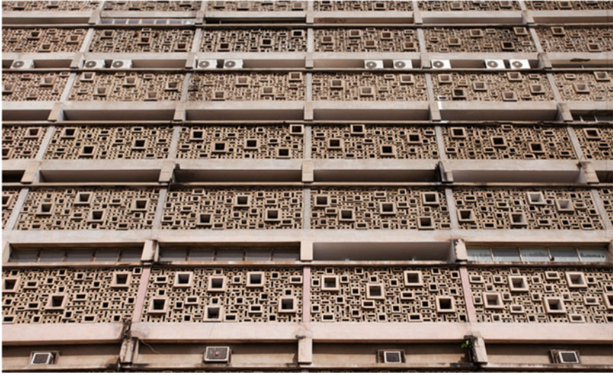
Fig. 5 Abreu, Santos and Rocha building in Maputo (1953–1956) designed by the architect Pancho Guedes. The shading of the loggias of the individual lodgings is resolved through a composition of brise-soleil which also allows ventilation ( Credits Forjaz 2011 )
