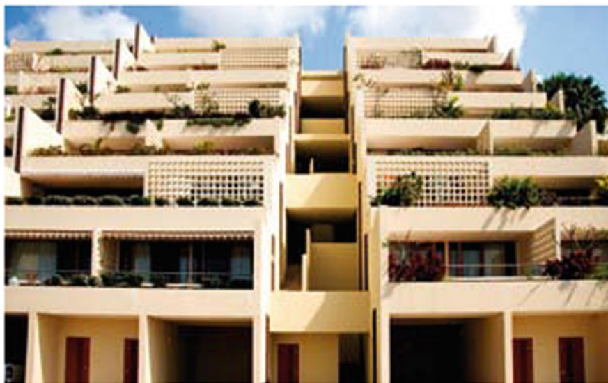
Fig. 4 Condominio do Caracal at Maputo. A residential building that include different strategies to limit overheating indoor. In particular, the most important strategies implemented are: Integration of planted areas on all exterior surfaces of the houses, an adequate orientation, the cross-ventilation, the shading device for the openings ( Credits Forjaz 2011 )
