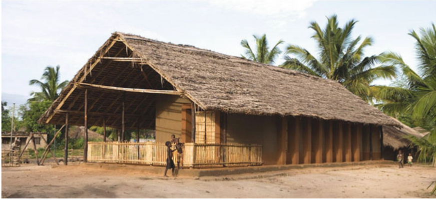
Fig. 7 A series of strategies combined in a single building, a school in Capo Delgado, in the northern part of Mozambique: massive masonry, a large roof to protect masonry and openings from solar radiation, large openings for natural ventilation, the presence of arcades for carry out part of the activities outdoors, light cover to allow micro-ventilation of the structure ( Credits ZRS Architekten Ingenieure, Photo Paula Holtz )
