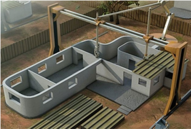
Fig. 1 Portal 3D printer with a robot manipulator [15]
