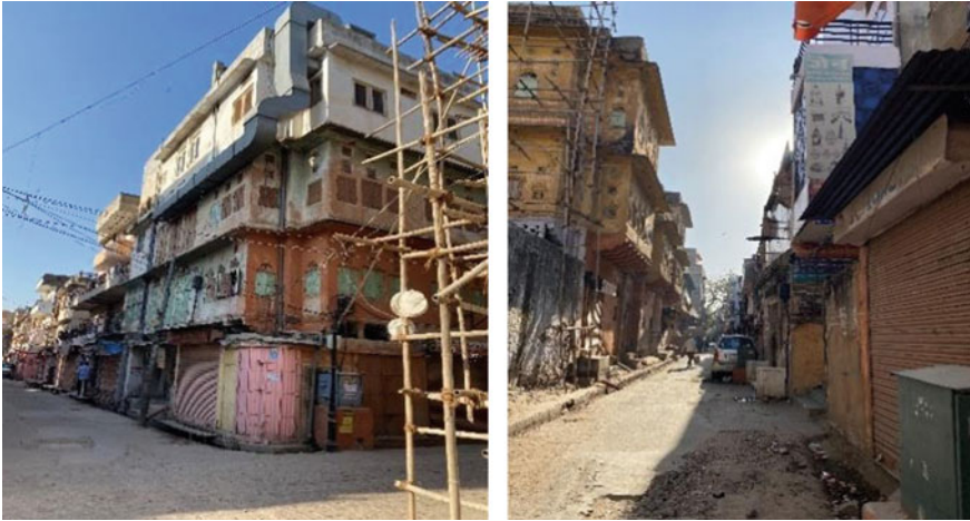
Fig. 7 Images showing new developments happening in walled city area without paying attention to the authenticity to cultural heritage
