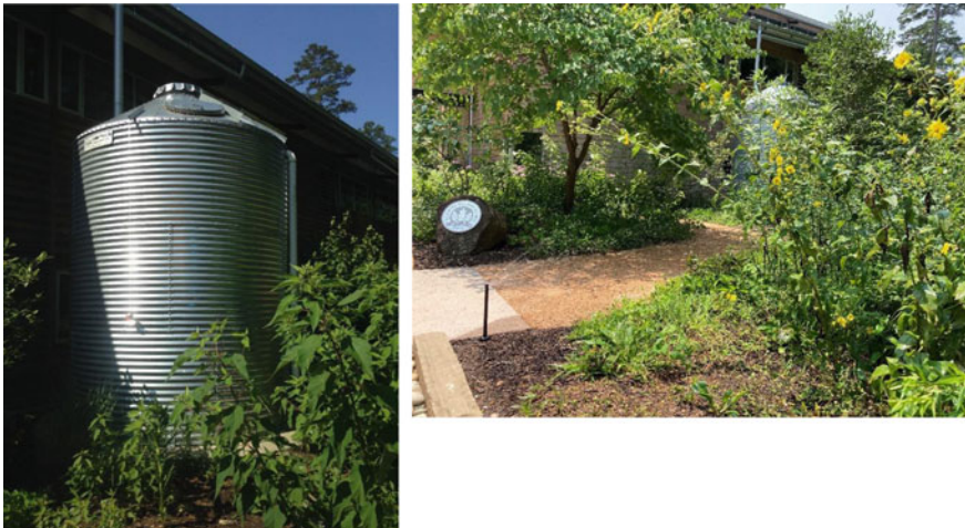
Fig. 3 (Left) One of the seven cisterns used to collect rainwater at the NC Botanical Garden at UNC-Chapel Hill (the one pictured is approximately 18,000 L). (Right) The sprinkler system connected to the RWH system that is used to irrigate the gardens. Photo courtesy of UNC-Chapel Hill
