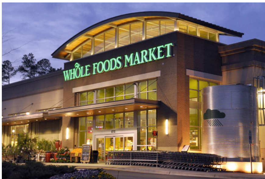
Fig. 5 The aboveground cistern, which is used for indoor toilet flushing, is prominently displayed at the entrance of the Whole Foods Market—the anchor store for the Market at Colonnade development (Photo courtesy of Regency Centers)
