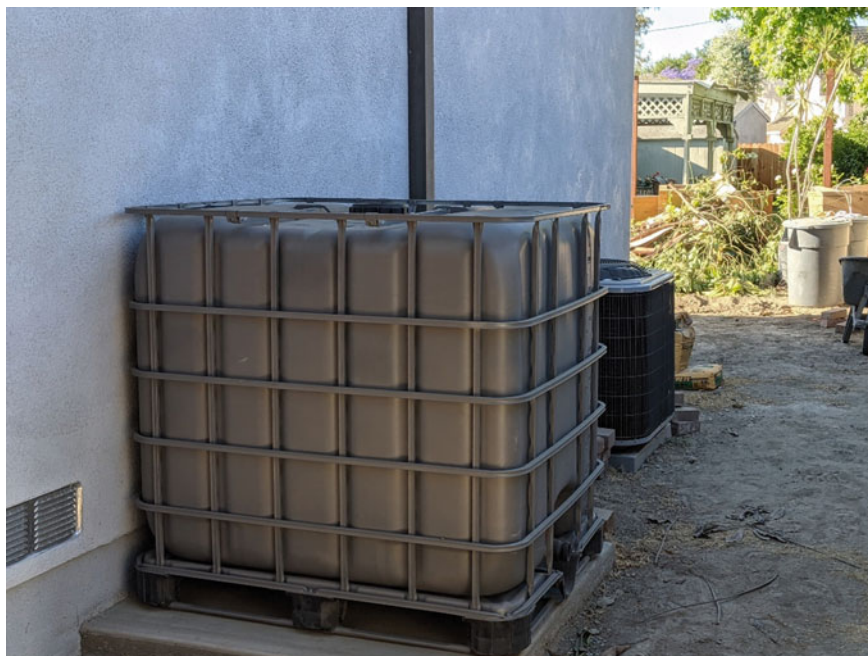
Fig. 1 Rain barrel in the city of Long Beach, CA (1,000 L; Courtesy of Dr. Suzanne Dallman, California State University Long Beach)
