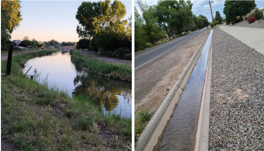
Fig. 12 A major canal extending from the Colorado River into the Grand Valley (left), a minor canal extending to individual parcels (right). Photos by author 2021
