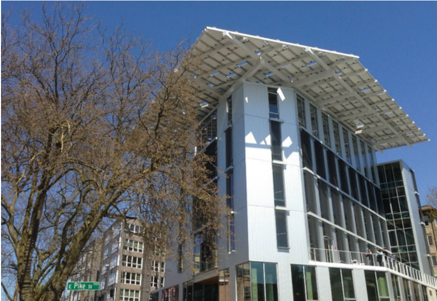
Fig. 1 The Bullitt Center (Seattle, WA) is a 6-story office building that houses approximately 170 tenants from a variety of businesses ( Source Phillip Thompson)
