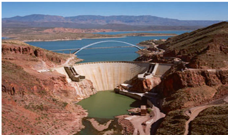
Fig. 6 Arch dam. (Source: Field Study, 2021)
