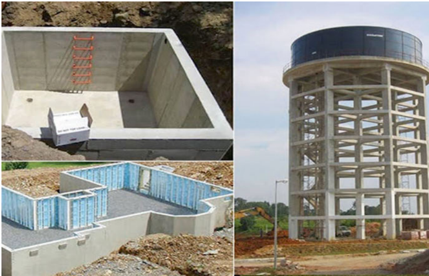
Fig. 11 Concrete materials for water retaining structures. (Source: Field Study, 2021)
