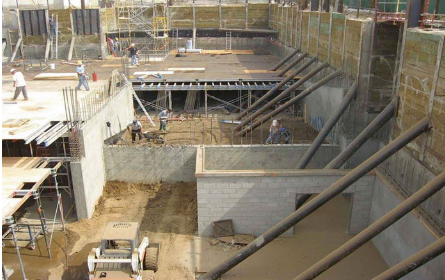
Plate 2 Ongoing construction works with emphasis on sustainable infrastructures. (Source: Field Study 2021)
