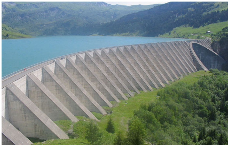
Fig. 5 Buttress dam. (Source: Field Study, 2021)
