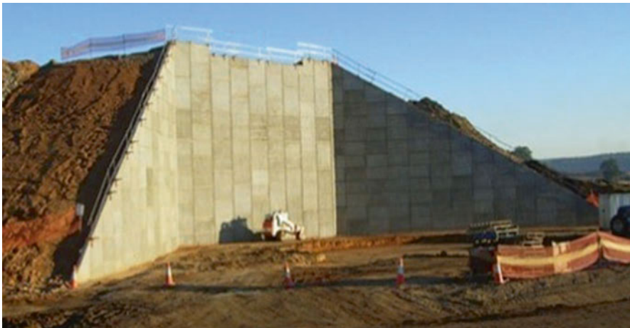
Fig. 2 Typical gravity retaining wall. (Source: Field Study, 2021)
