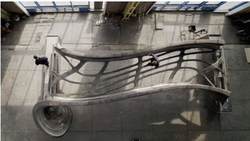
Fig. 3 MX3D smart bridge under construction (photo © Joris Laarman Lab)
