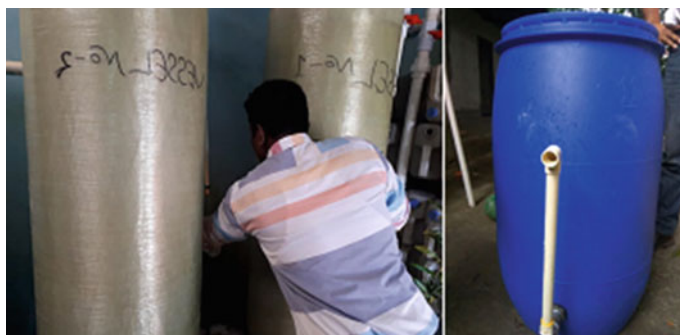
Fig. 6 Community scale and household scale adsorption bed with arsenic removal media
