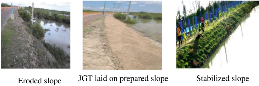
Fig. 56.5 Application of JGT for slope stabilization of road of embankment
