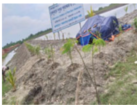
Preparation of slope
