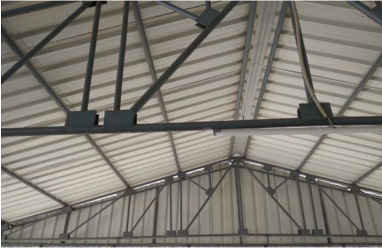
Fig. 71.5 King post truss with gussets
