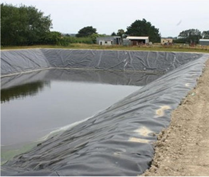
Fig. 34.4 High-density polythene lining
