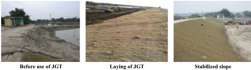
Fig. 56.1 The jute geotextile for reconstruction of embankment damaged by cyclone
