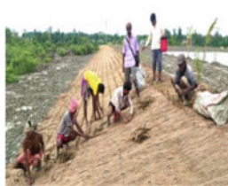
Laying of JGT
