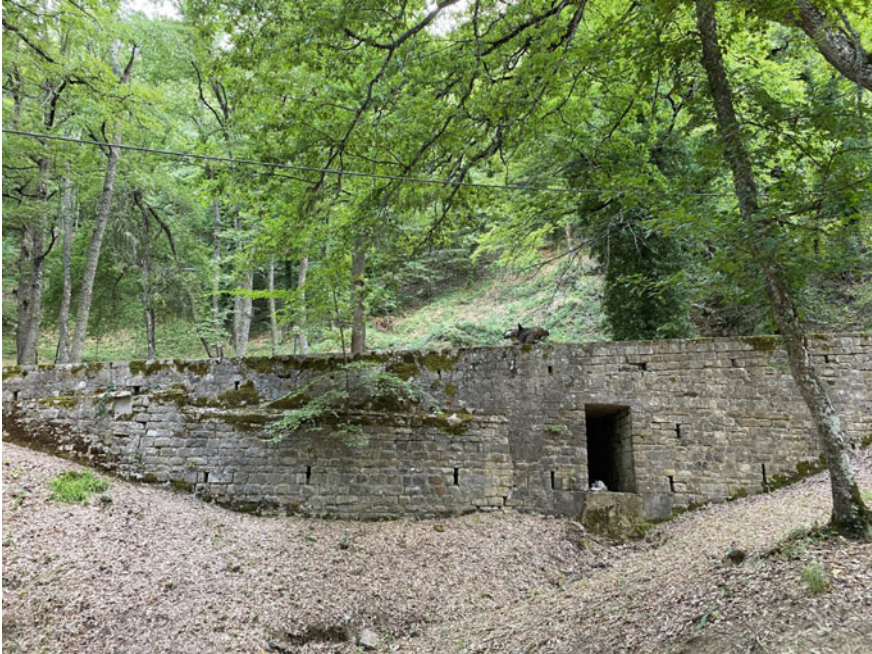
Fig. 51.17 Hydraulic interventions to reduce soil erosion by means of small sedimentation weirs. Source Interregional River Basin Authority of Basilicata
