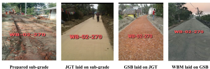
Fig. 56.2 The woven jute geotextile for strengthening weak road sub-grade
