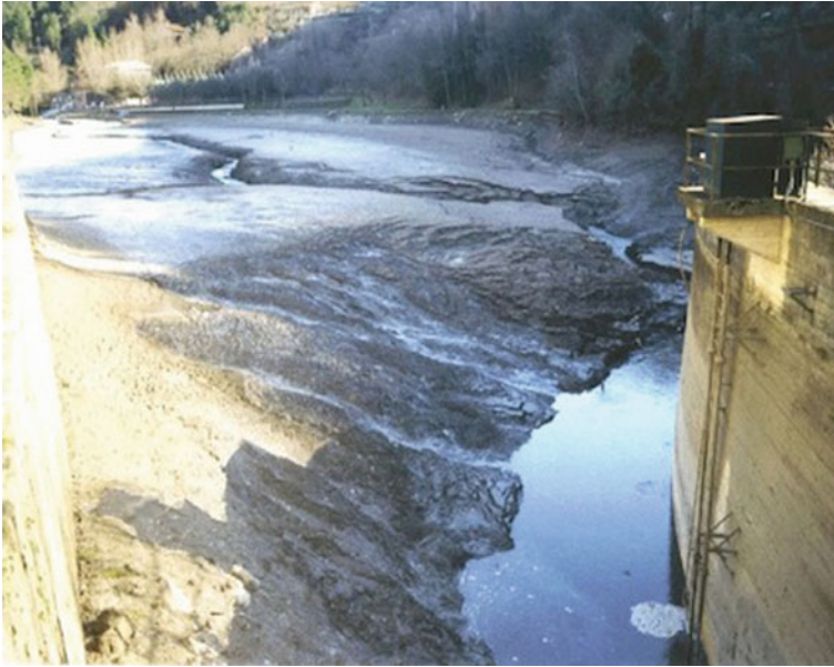
Fig. 51.13 Accumulation of sediments in reservoir. Source Interregional River Basin Authority of Basilicata
