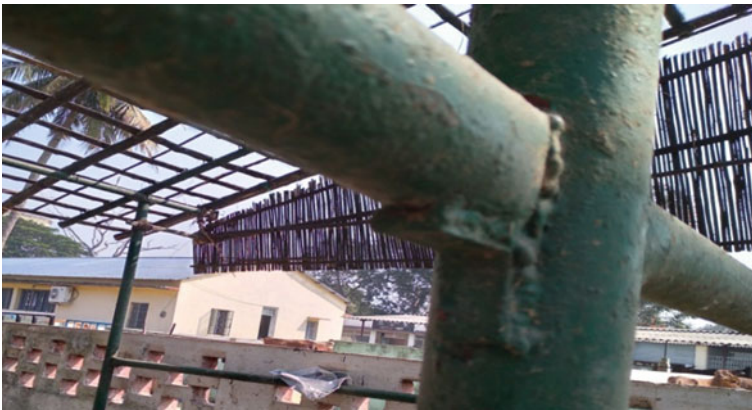
Fig. 71.6 Iron frame with metal strap-L clamp
