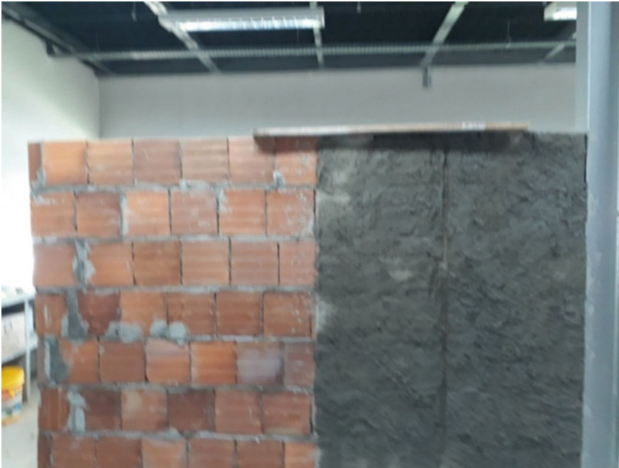
Fig. 5 Wall of ceramic blocks with plaster being applied
