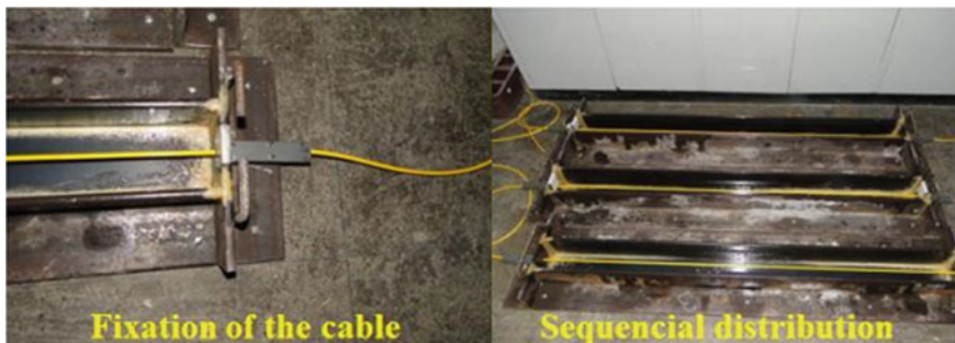
Fig. 22 Installation of the sensors in the molds (Rocha et al. 2013)
