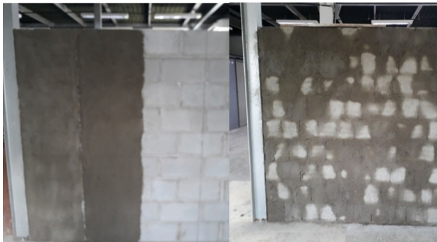
Fig. 6 Concrete and ceramic block walls with roughcast containing lime
