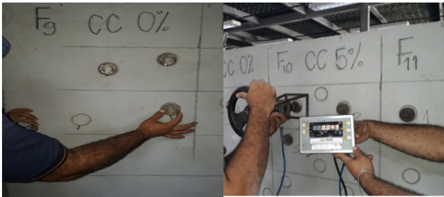
Fig. 9 Gluing the adhesion plates and Adhesion test
