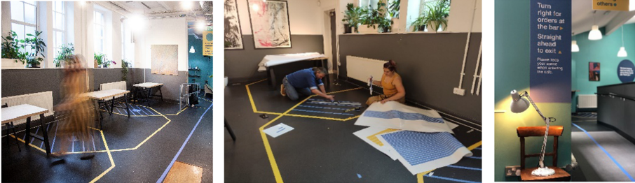
Fig. 3. Installation of the signage in the Storey building, Lancaster, UK.
