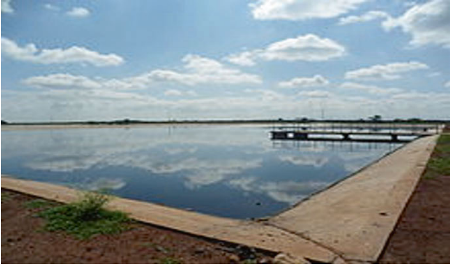
Fig. 10.2 A lagoon used for biological treatment of wastewater (Facultative Lagoon 2021 )
