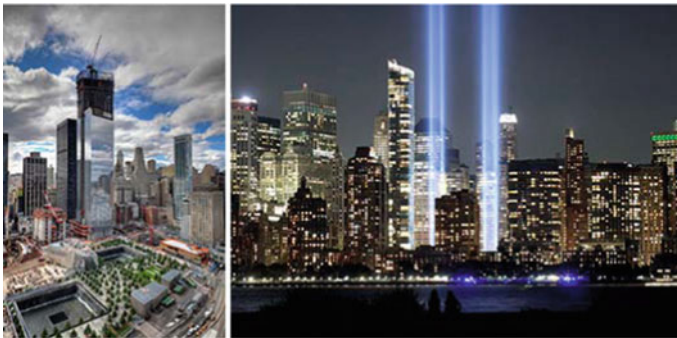
Fig. 3 Twin Towers in New York. The use of the site of improvement in place of the towers
