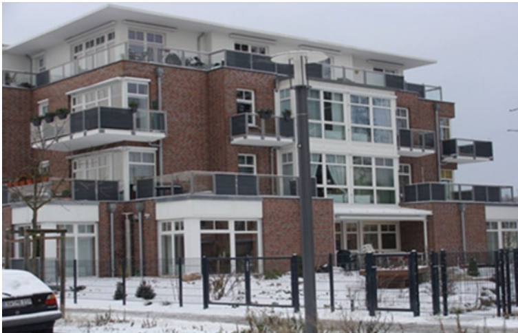
Fig. 4 Arranging developed (glazed and open) summer rooms for each individual apartment. Berlin, city villa
