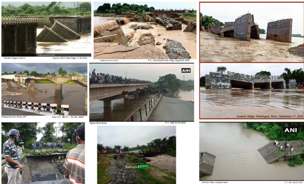
Fig. 11.8 Examples of bridge failures during the monsoon of 2020 from different parts of India ( Source Collected by author from various electronic media mentioned below in each photo)
