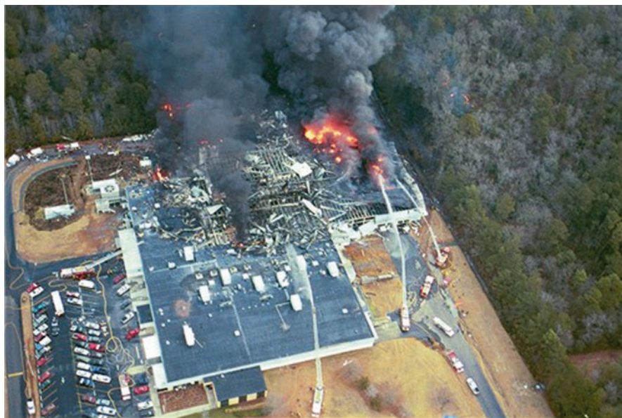
Fig. 10.22 Fire following explosions at West Pharmaceutical Services, Inc., Kinston, NC, USA. (Source: U.S. Chemical Safety Board, 2003)
