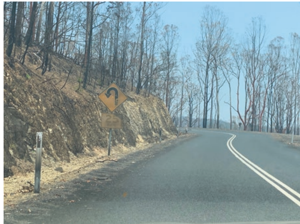
Fig. 7.7 After bushfire. Armidable Road, Clouds Creek, NSW. (Photo is taken on January 4, 2020. ©Photo by Elena Filkova, used with permission)
