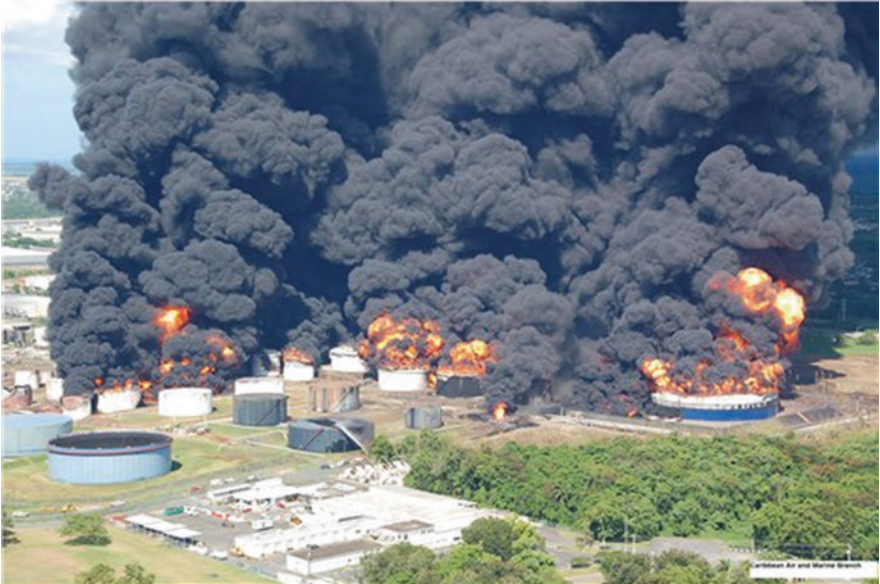
Fig. 1.1 Aerial view of October 23, 2009 fire, Caribbean Petroleum Investigation. (Source: https://www.csb.gov/caribbean-petroleum-investigative-photos . Accessed July 2020)
