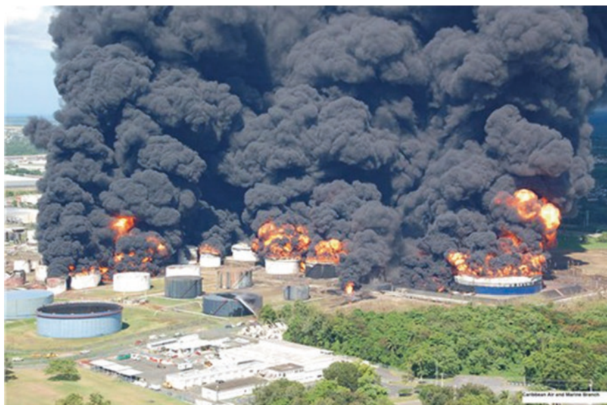
Fig. 10.25 Fire at Caribbean Petroleum Corporation Tank Terminal, Bayamon, Puerto Rico, USA. (Source: U.S. Chemical Safety Board, 2015, courtesy U.S. Customs and Border Protection, Caribbean Air and Maritime Branch)
