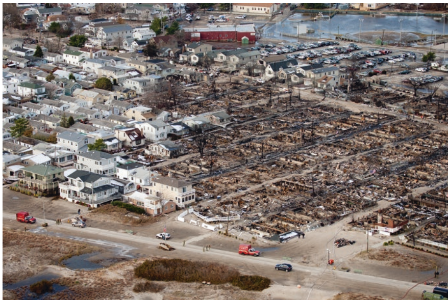
Fig. 13.17 Aerial view of flood and fire damage caused by Hurricane Sandy, Breezy Point Neighborhood, Queens, NY, 2012. (Source: US FEMA, Andrea Booher)
