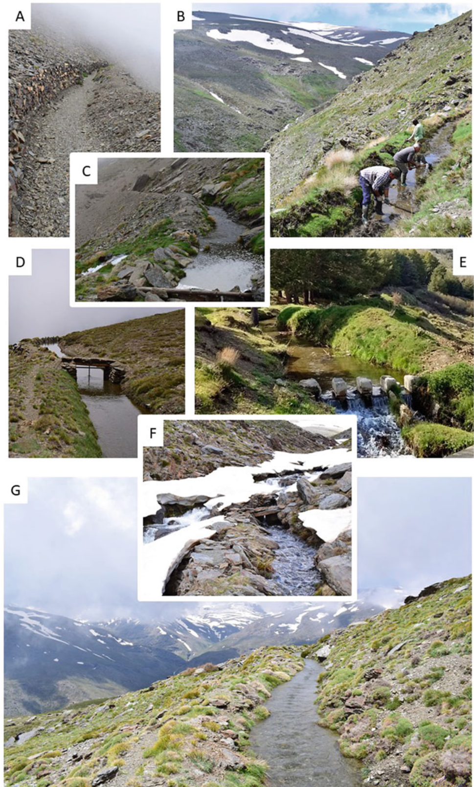
Fig. 1 a Acequia de careo without water to carry out repair works. b Members of Bérchules' irrigation community cleaning an acequia de careo . c Aliviadero on the side. d Aliviadero overflow and flow limiter. e Partidor of acequia de careo of the Poqueira ravine. f Water catchment for an acequia de careo . g Acequia de careo of Bérchules
