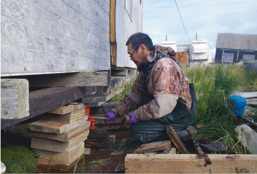
Fig. 10.3 Savoongan whaler and walrus hunter props up his house as it sinks into the melting permafrost. (Source: Parlow © 2019)
