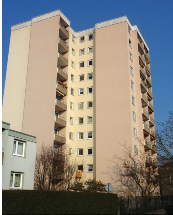
Fig. 35.2 Eleven-story high-rise building with a cable-driven elevator
