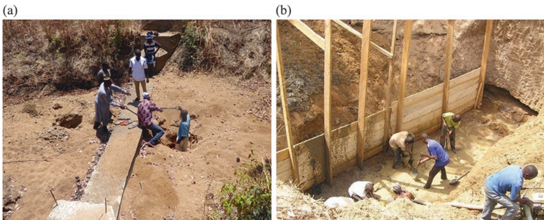
Fig. 5.13 (a) Sand dam construction nearing completion (b) during construction
