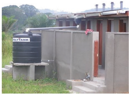
Fig. 5.15 Kumasi Ventilated Improved Pit or KVIP with hand washing facility
