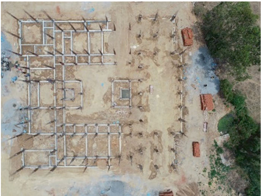
Fig. 57.9 Boys hostel at Mohan kumaramangalam medical college at Salem
