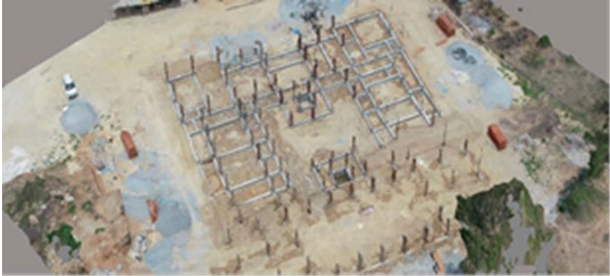
Fig. 57.19 3D Image of Additional building site processed in context capture
