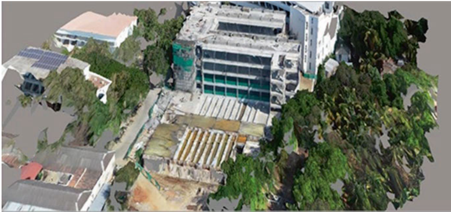
Fig. 57.12 3DImage of Arts block Processed in Context capture
