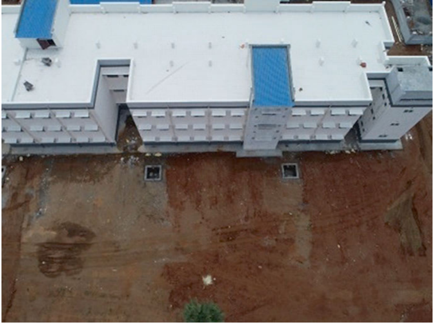
Fig. 57.8 Additional supports building at Krishnagiri
