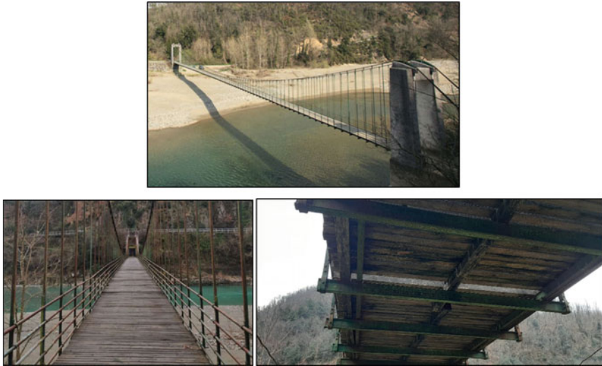
Fig. 1 Different views of the footbridge
