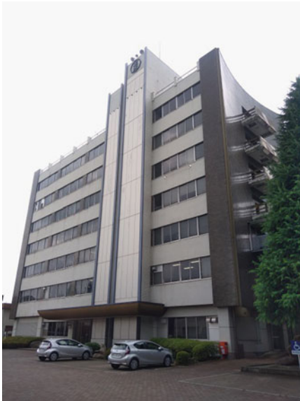
(a) Seven story RC building
