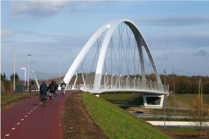
Fig. 1 Bicycle bridge Tegenbosch [13]
