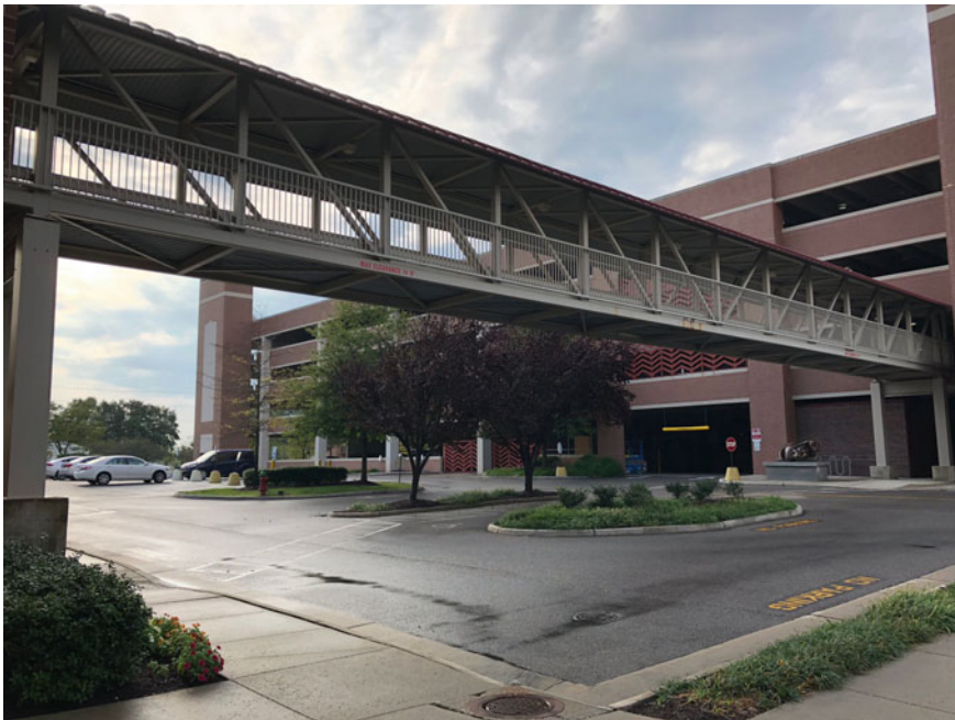
Fig. 1 Side view of the footbridge
