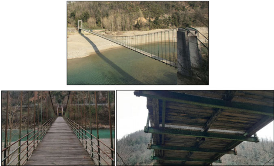
Fig. 1 Different views of the footbridge
