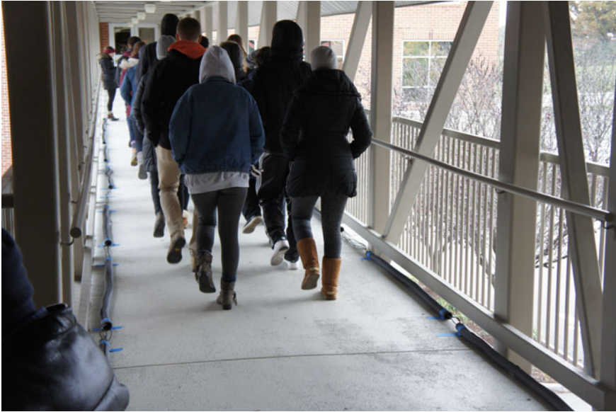
Fig. 3 Volunteers walking across the footbridge
