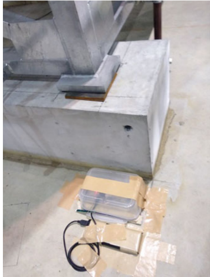
(b) Sensor unit on Roof floor
