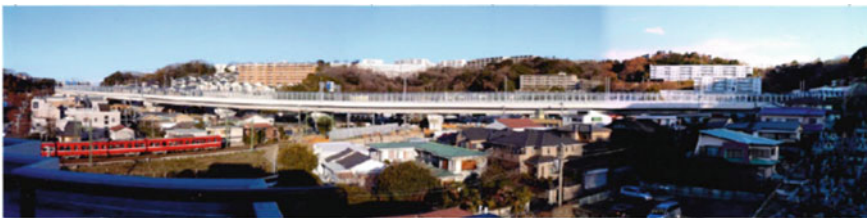
Fig. 1 Panoramic view of the study bridge structure
