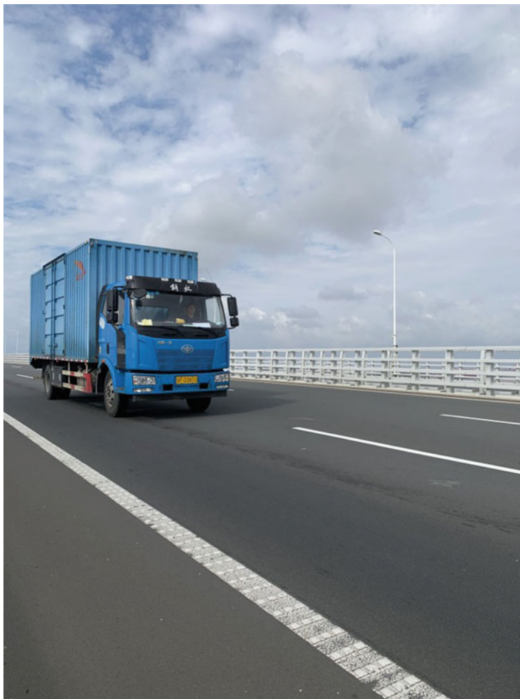
Fig. 10 Truck passed through the Chongqi bridge
