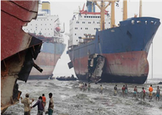
Fig. 18.1 Beaching method. Reprinted with permission from Elsevier [8]
