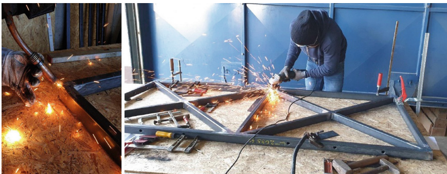
Fig. 17. Supporting structure welding and grinding.
