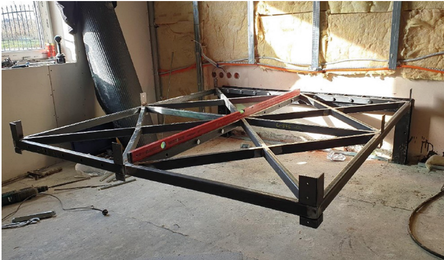
Fig. 16. Supporting structure montage.
