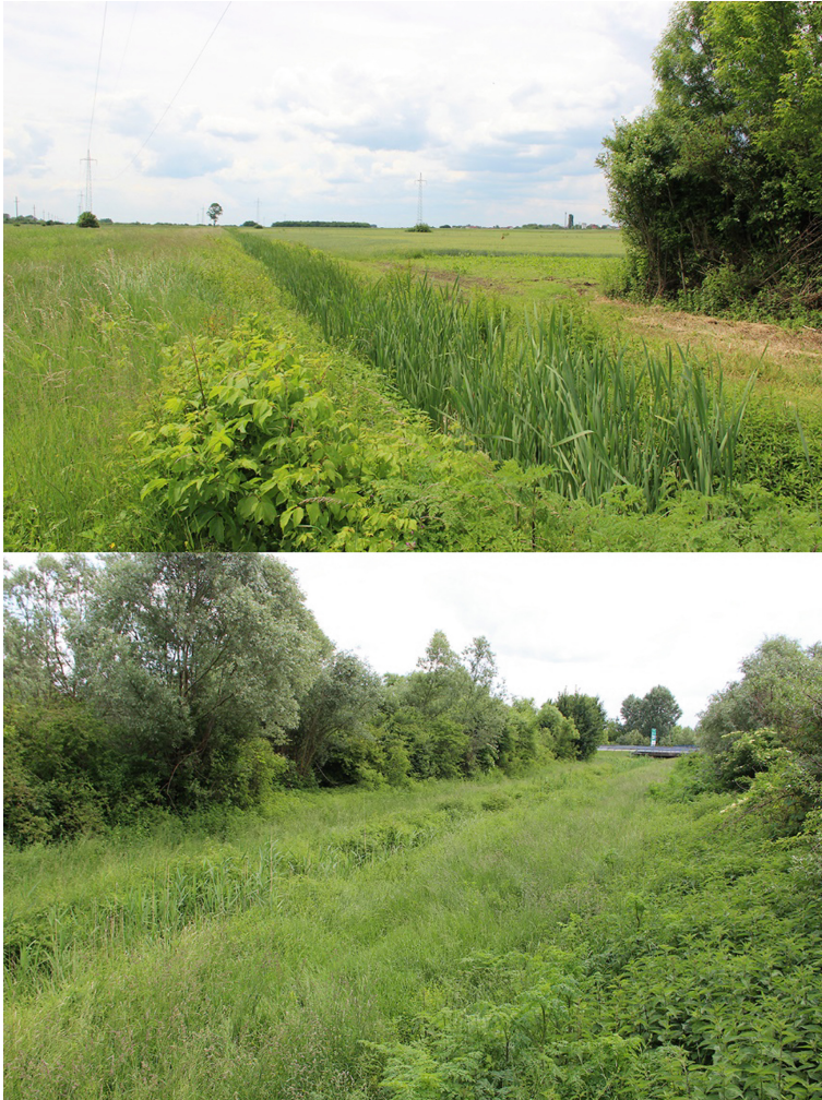
Fig. 4. The state of overgrowth with swamp vegetation of one of the detailed channels of the Krčevina field drainage (upstream view), and the Topolovac receiver (view towards the highway downstream) in the spring of 2020.
