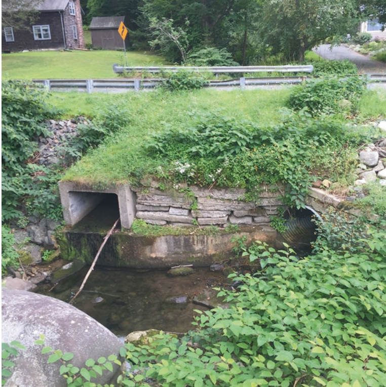
Fig. 5.8 Existing roadside culverts. (Courtesy of Nitsch Engineering)
