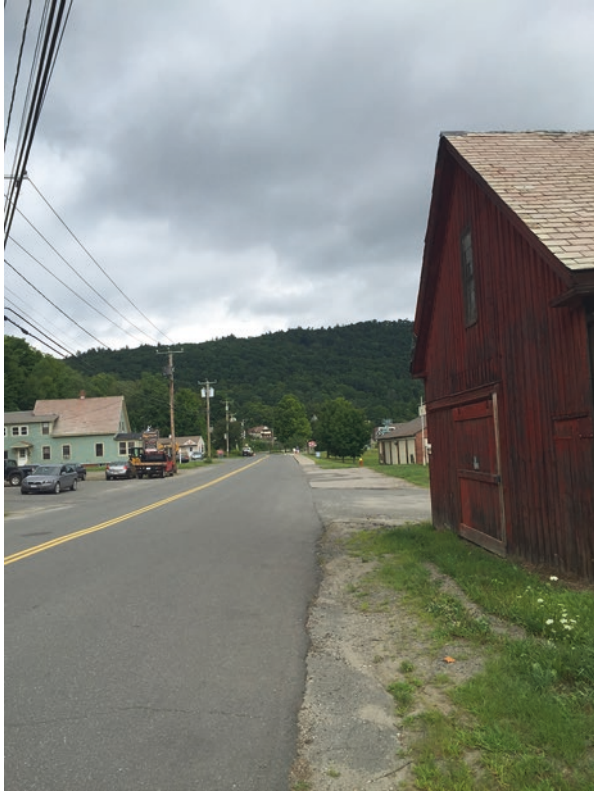
Fig. 5.7 Edge of road and sidewalk connectivity issues. (Courtesy of Nitsch Engineering)
