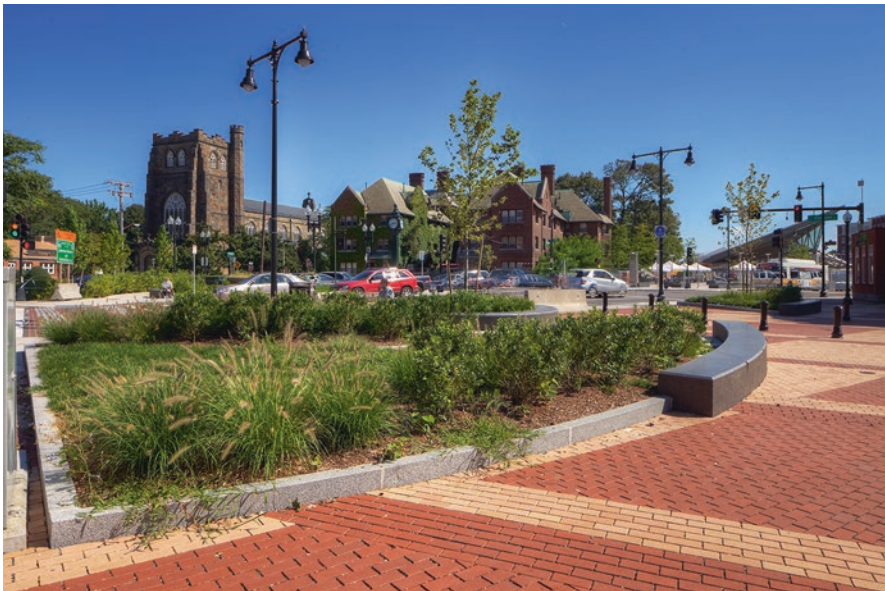
Fig. 5.3 Peabody Square landscaping includes bioretention, rain gardens, pervious pavers, and aesthetic improvements. (Courtesy of Nitsch Engineering)
