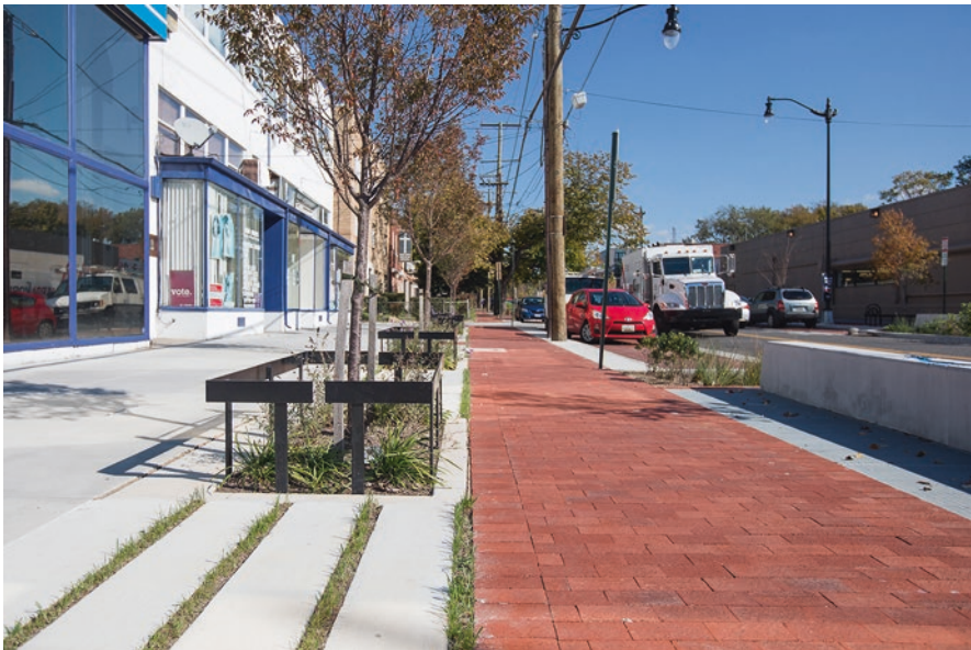
Fig. 5.5 Landscape infiltration gaps on Kennedy Street. (Courtesy of Nitsch Engineering)
