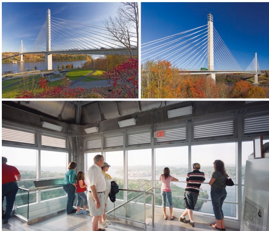
Fig. 9.22 The 2120'-long Penobscot Narrows Bridge and Observatory in Maine features a 1161' main span and the world's tallest public bridge observatory at 420'. Horizontal articulations were recessed into the pylon as it was built giving the impression of large stone while at the same time hiding the construction joints. (Courtesy of FIGG)
