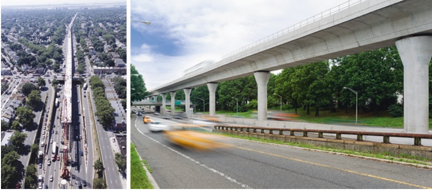
Fig. 9.5 AirTrain JFK consists of nine miles of elevated rail transit that carries passengers into JFK International Airport in New York. (Courtesy of FIGG)
