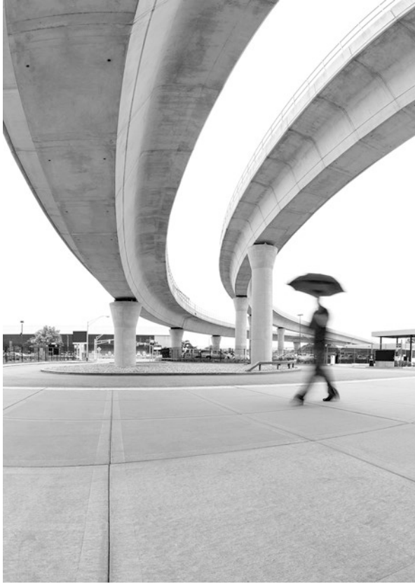
Fig. 9.14 AirTrain JFK consists of nine miles of elevated rail transit that carries passengers into JFK International Airport in New York. Consistent single sourcing of materials creating the concrete mix design results in a natural uniform color. (Courtesy of FIGG)
