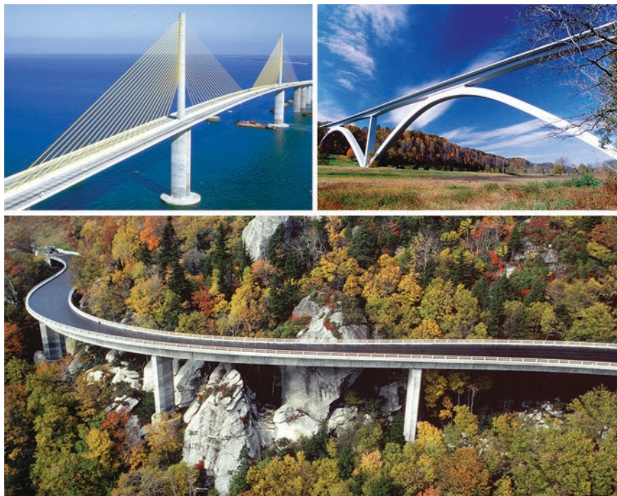
Fig. 9.1 Winners of three Presidential Design Awards through the National Endowment for the Arts. Only five of these awards for bridges were ever given by the presidents of the United States (left to right): I-275 Bob Graham Sunshine Skyway Bridge (Florida), Natchez Trace Parkway Arches (Tennessee), and Blue Ridge Parkway Viaduct (North Carolina). (Courtesy of FIGG)
