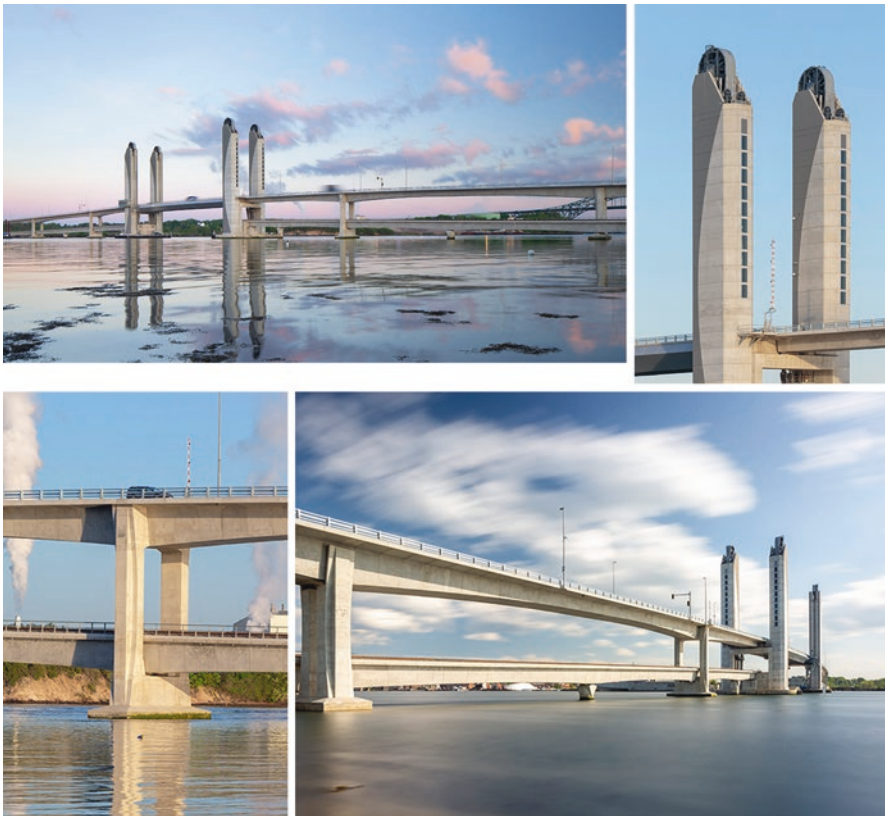
Fig. 9.23 The Sarah Mildred Long Bridge carries US Route 1 Bypass and a heavy rail line that serves the Portsmouth Naval Shipyard over the Piscataqua River. Sculptural shapes with long open spans open new vistas. (Courtesy of FIGG)
