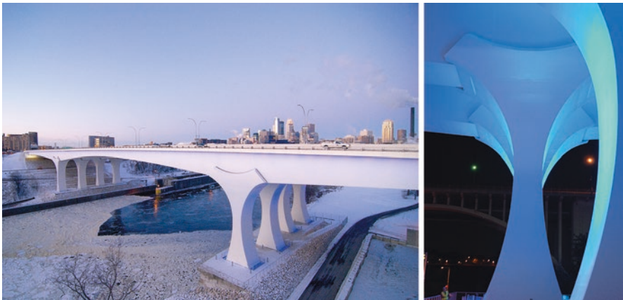
Fig. 9.21 The New I-35W Bridge in Minnesota was designed and built in 11 months with a 504' precast concrete segmental main span across the Mississippi River. Nanotechnology concrete, which is a material that cleans pollution from the air, was used for gateway sculptures. (Courtesy of FIGG)
