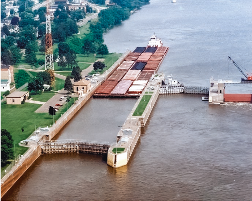
Fig. 10.8 Typical 15-barge tow at Lock and Dam 12, Mixed Cargo, Mississippi River. (Courtesy of US Army Corps of Engineers, Rock Island District)
