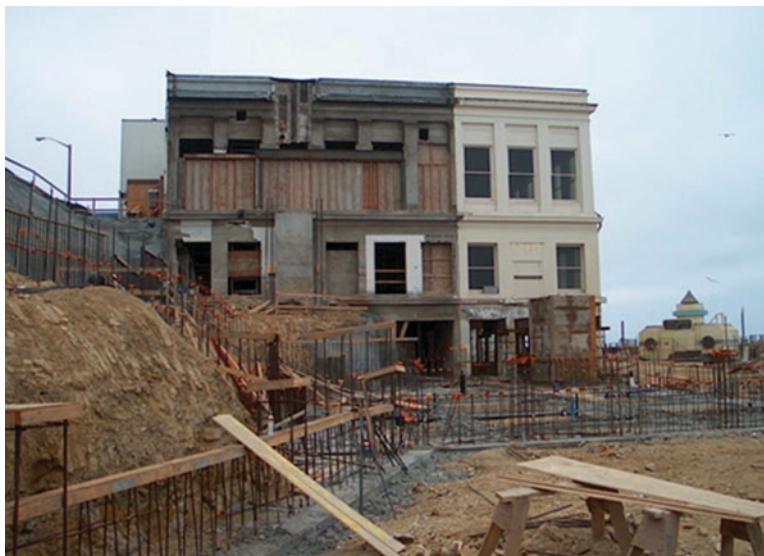
Fig. 19.2 Cliff House construction, second phase. (Courtesy of Project Architect Carrie Strahan)
