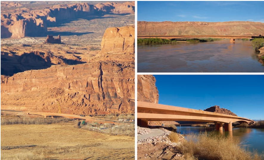
Fig. 9.13 The US 191 bridges over the Colorado River blend seamlessly with the spectacular landscape of Utah’s Canyonlands region fulfilling the community’s vision of “A Bridge in Harmony with the Environment.” (Courtesy of FIGG)
