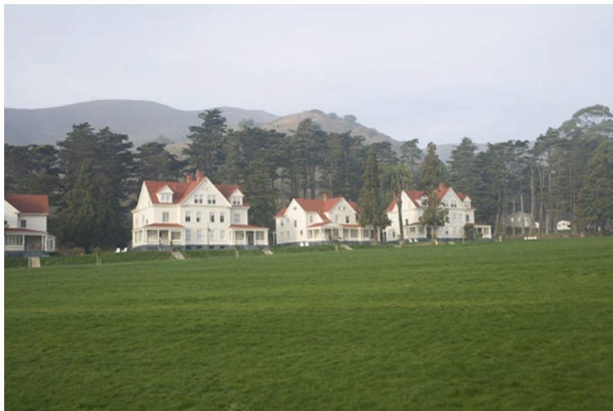
Fig. 19.4 Rehabilitated historic buildings, now part of Cavallo Point Lodge, and parade ground. (Courtesy of Project Engineer Melanie Wollenweber)
