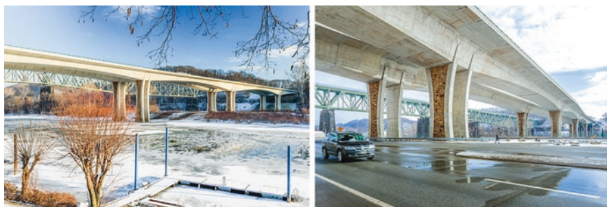
Fig. 9.7 The I-76 Allegheny River Bridge is Pennsylvania's longest concrete span at 532' and provides an environmentally friendly river crossing. The texture and color on the piers reflect the rock layers in the embankments leading up to the bridge and the stonework in the adjacent Oakmont Country Club. (Courtesy of FIGG)
