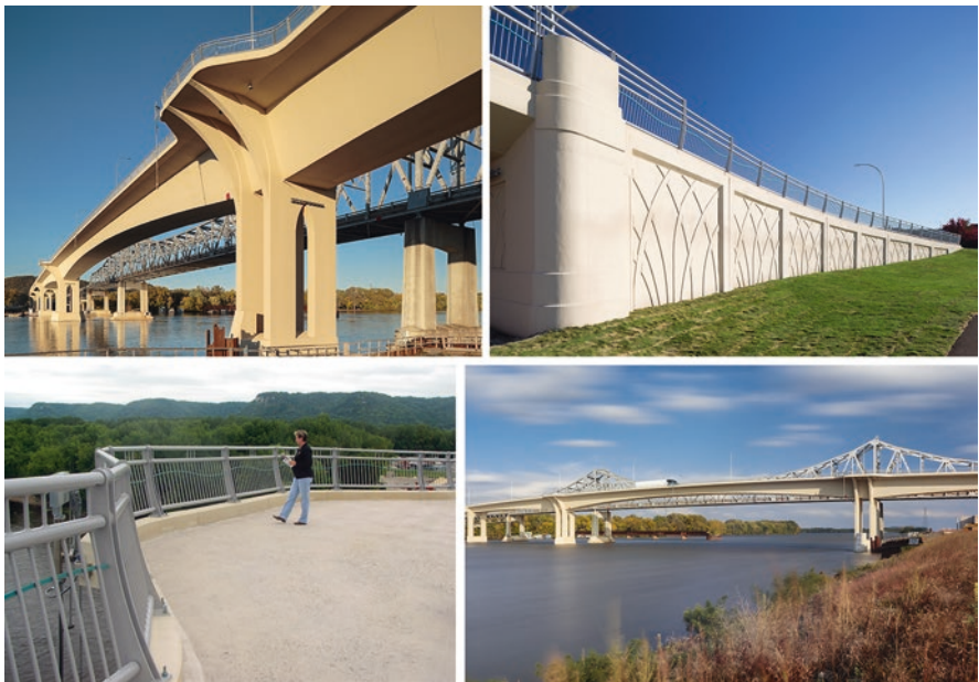
Fig. 9.16 Winona Bridge. Context-sensitive aesthetic features of the Winona Bridge in Minnesota celebrate the organic beauty of the Mississippi River and preserve the historical importance of the existing bridge. (Courtesy of FIGG)
