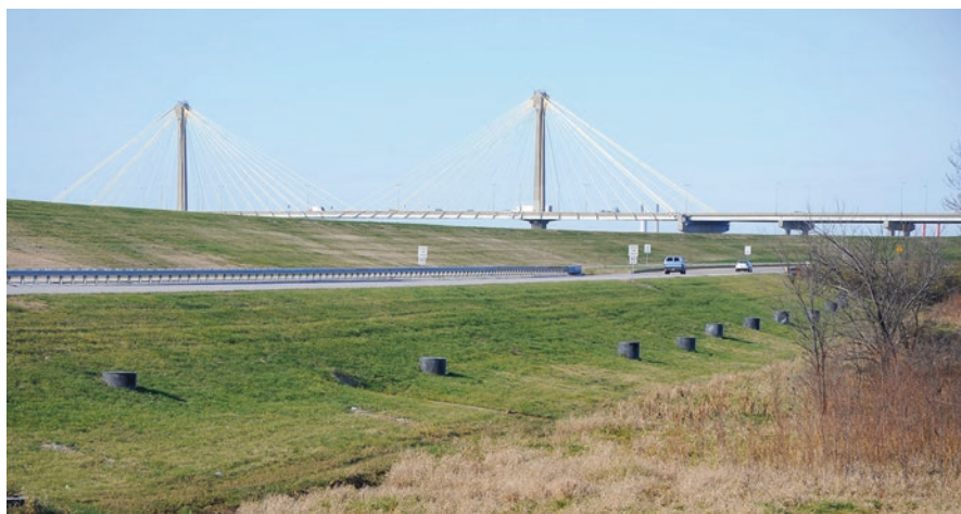
Fig. 14.1 Example of a typical earthen levee embankment, Upper Wood River Levee System, Illinois. (Source: USACE)
