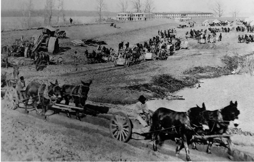
Fig. 14.2 Early levee construction along the Mississippi River. (Source: USACE)
