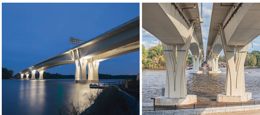
Fig. 9.10 The I-90 Dresbach Bridge features a 508'-long main span over the Mississippi River that was built from above while maintaining commercial and recreational river traffic during construction. Piers are sculpturally designed to pay tribute to the old-growth trees. (Courtesy of FIGG)
