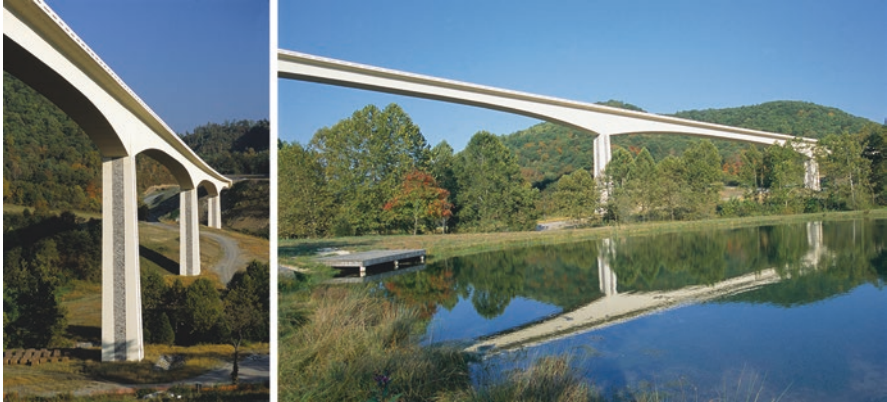
Fig. 9.15 Smart Road Bridge. Preservation of the rural beauty of the Ellett Valley made aesthetics a major focus of the Smart Road Bridge in Blacksburg, Virginia. Long, sweeping, curved spans enhance openness in the natural setting. Use of Hokie Stone on the piers connects the bridge to the native material of the hillsides. (Courtesy of FIGG)
