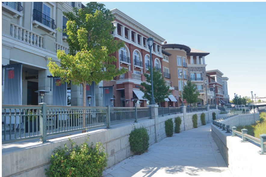
Fig. 14.4 A view of a terraced floodwall that also serves as a walking path along the Napa River in California. (Source: USACE)
