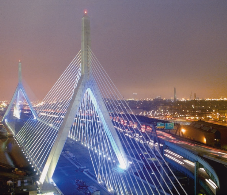
Fig. 9.17 The I-93 Leonard P. Zakim Bunker Hill Bridge was the widest cable-stayed bridge in the world at 183' with ten lanes when it was completed. The lighting of the pylon legs brings to life the bridge shape and gateway design at night. (Courtesy of FIGG)
