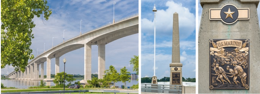
Fig. 9.3 New Jersey’s Victory Bridge. The Victory Bridge features a record-setting 440’-long precast concrete segmental main span over the Raritan River in New Jersey and pays tribute to WWI Veterans with a series of bronze plaques recognizing US Marines, US Navy, US Army, Air Corps, and Red Cross. (Courtesy of FIGG)
