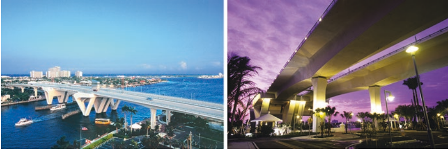
Fig. 9.8 The 17th Street Bridge in the busy Las Olas area of Fort Lauderdale, Florida, rises above the riverbanks and creates park spaces in the urban area below. Space is opened up below the bridge with long variable depth spans and slender sculptural piers. (Courtesy of FIGG)
