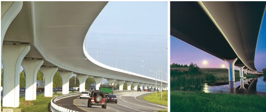
Fig. 9.4 The Selmon Expressway in Tampa, Florida, consists of 5.13 miles of elevated highway built in the median of the existing expressway using sculpturally shaped piers that are 6’ wide. (Courtesy of FIGG)
