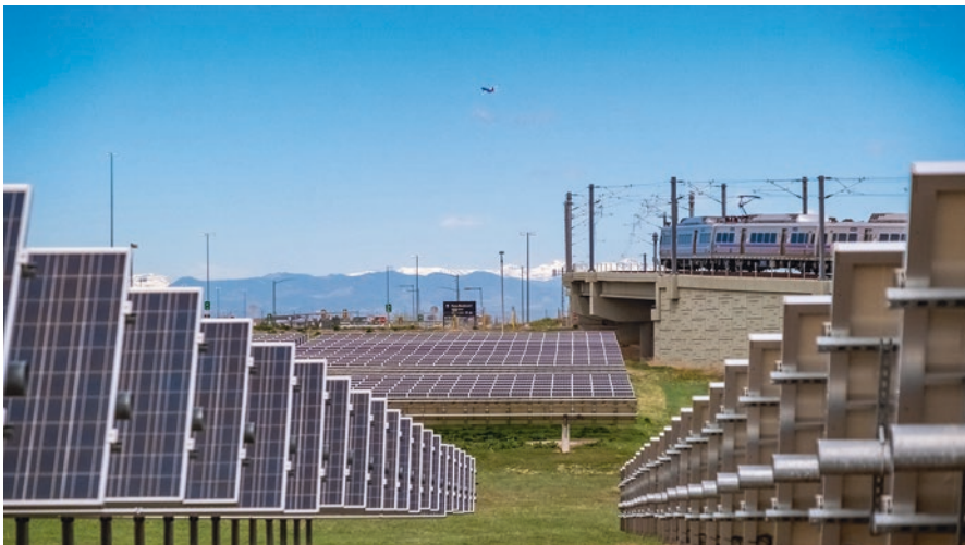
Fig. 4.2 DEN solar power array. (Courtesy of Denver International Airport)
