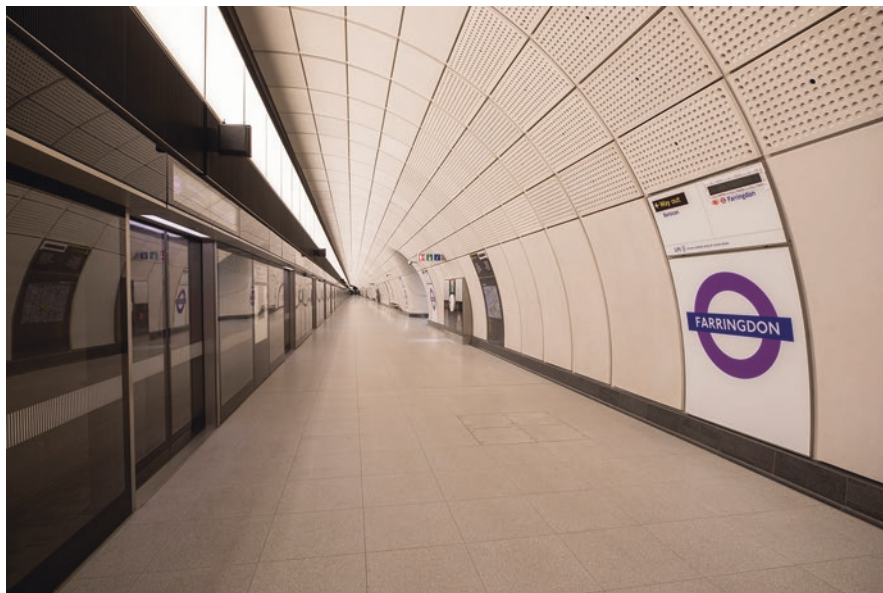
Fig. 12.23 The Elizabeth line, a modern London rail line, was built by Crossrail at a cost of $500M per mile. (Source: Crossrail Ltd.)
