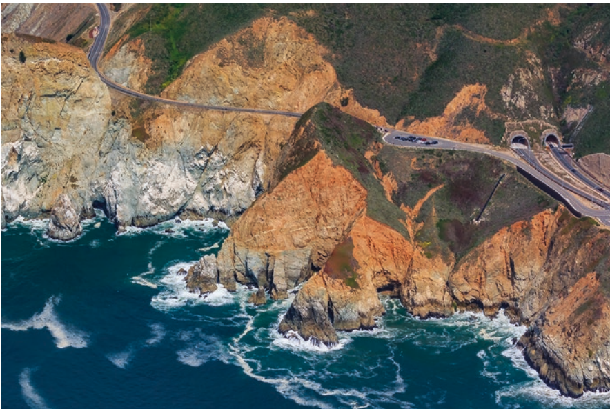
Fig. 12.12 Devil's Slide Tunnel portal on Route 1, in California. (Source: HNTB)
