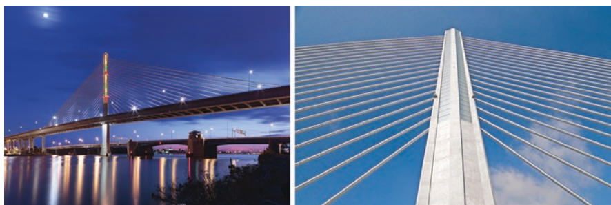
Fig. 9.24 The I-280 Veterans' Glass City Skyway in Toledo, Ohio, pays tribute to the area's rich heritage in the glass industry. (Courtesy of FIGG)
