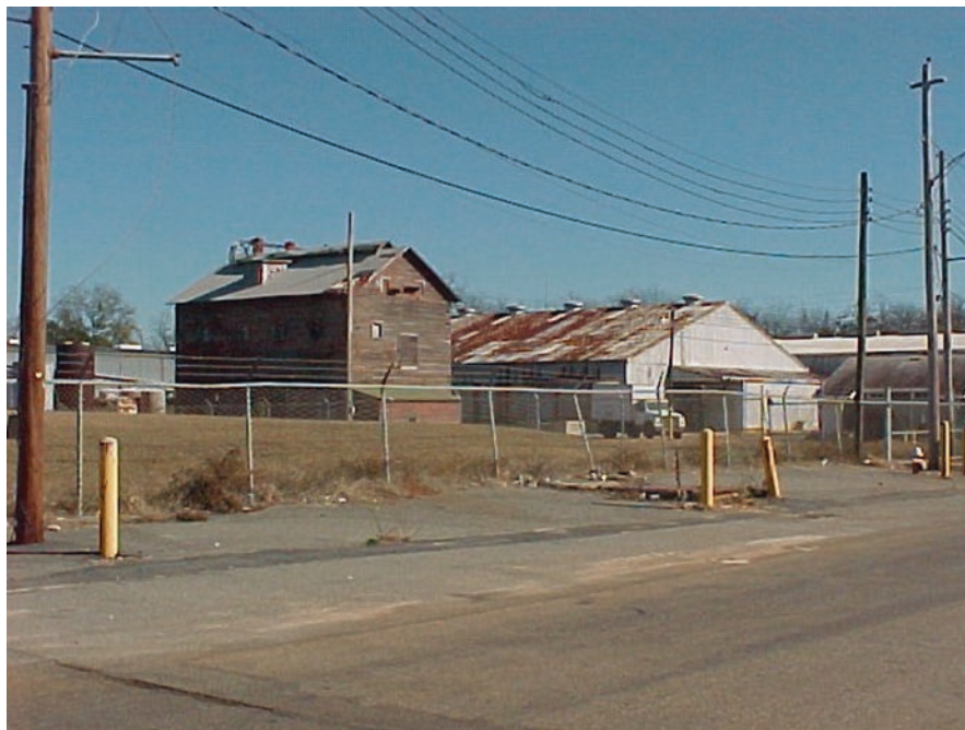
Fig. 15.6 The facility was used for almost 90 years for formulating and/or packaging pesticides, herbicides, and insecticides
