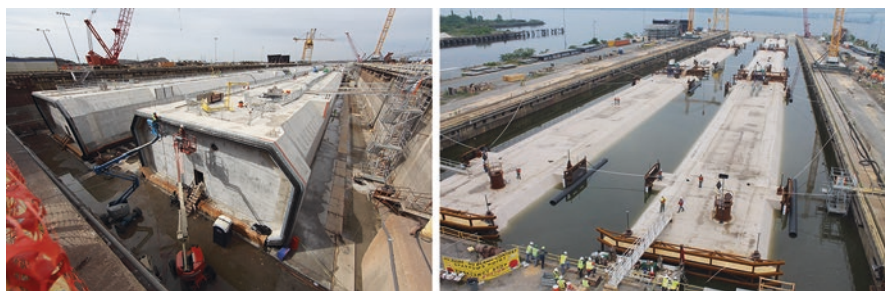
Fig. 12.19 Virginia’s Midtown Tunnel immersed tube construction. (Source: Tunneling Journal)
