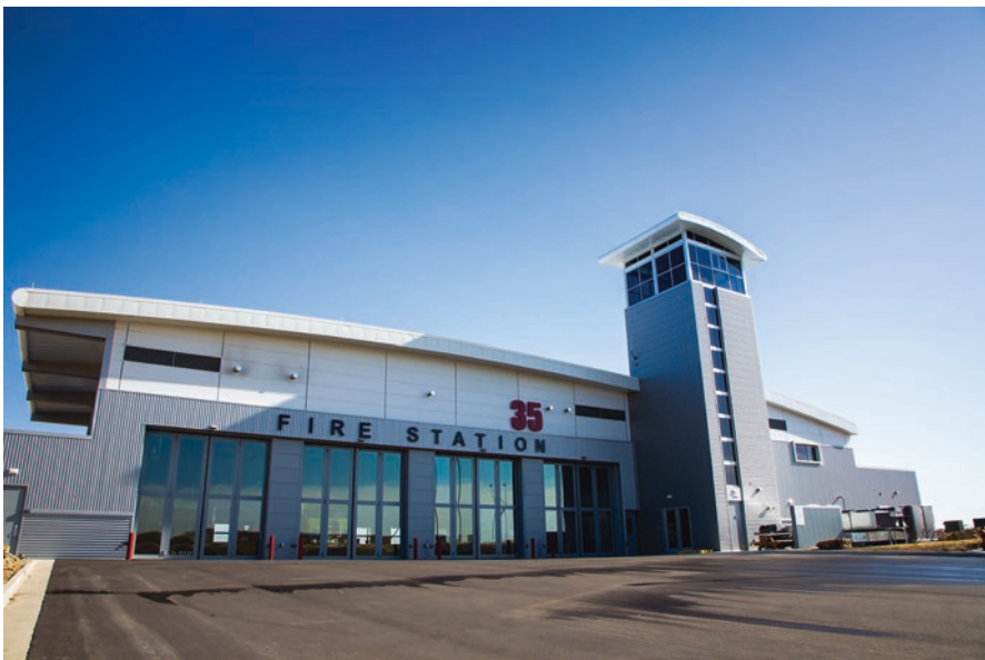
Fig. 4.4 DEN fire station. (Courtesy of Denver International Airport)
