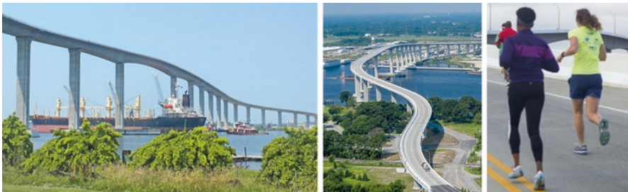
Fig. 9.6 The South Norfolk Jordan Bridge in Virginia is a 5375'-long high-level fixed bridge that keeps rail, vehicular, pedestrian, and maritime traffic moving at all times. (Courtesy of FIGG)
